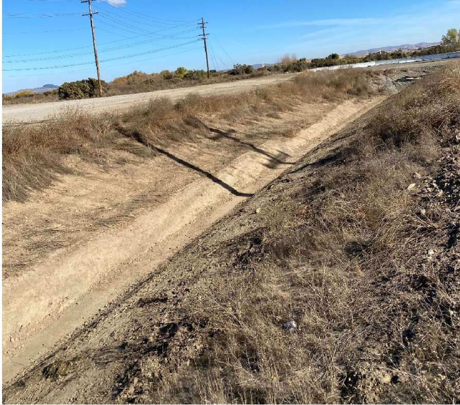
Photograph 7: Constructed swale located in the southern portion of the project site, drains into culvert, facing northeast
