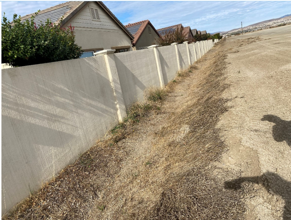
Photograph 1: Constructed swale along the western perimeter of the project site, facing north
