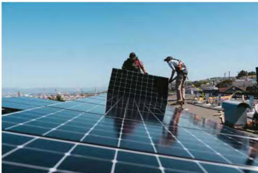
Workers install solar panels at a home in San Francisco, California. Photograph by Michaela Vatcheva / Bloomberg / Getty
