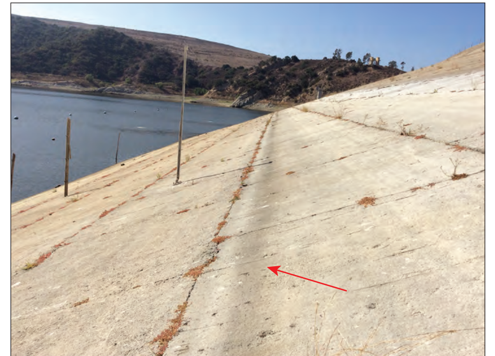
Photo 24: Ordinary High Water Mark is indicated by staining on the existing dam embankment. October 21, 2020.
