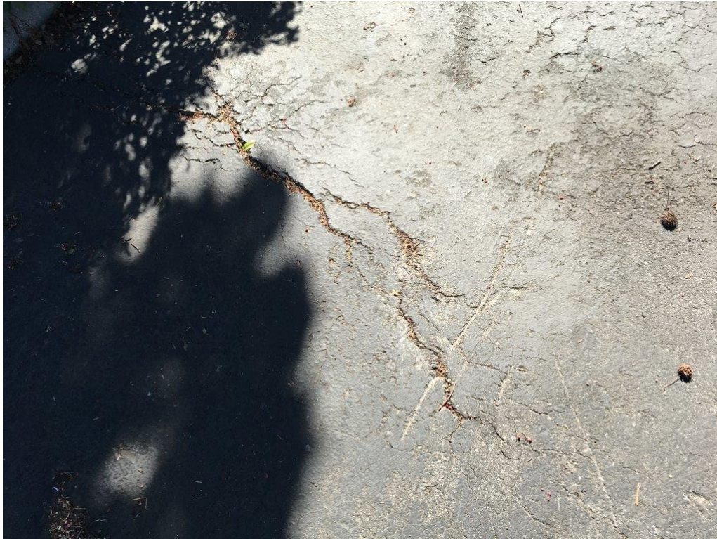
Photo 9: View of minor cracks in the asphalt-paved parking area in the central portion of the site.
