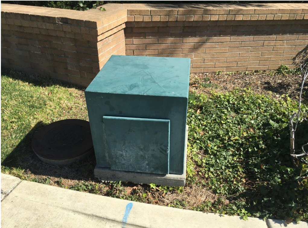
Photo 7: View of an unlabeled pad-mounted transformer along the northwestern site boundary.
