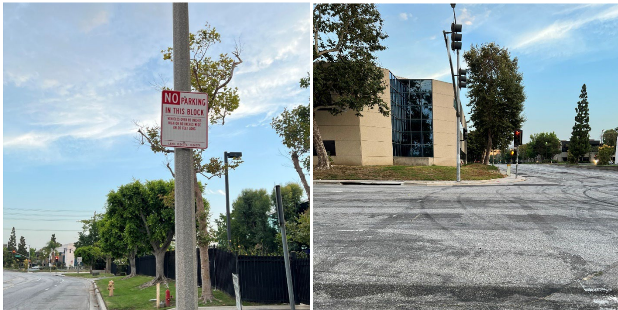
Large vehicle parking restriction, Via Oro Avenue southbound at Carson Street. Crosswalk at Via Oro Avenue and Carson Street (Photo Credit: Fehr & Peers, July 2023).
