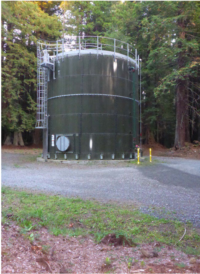
Existing Glass-Fused Bolted Steel Tank
