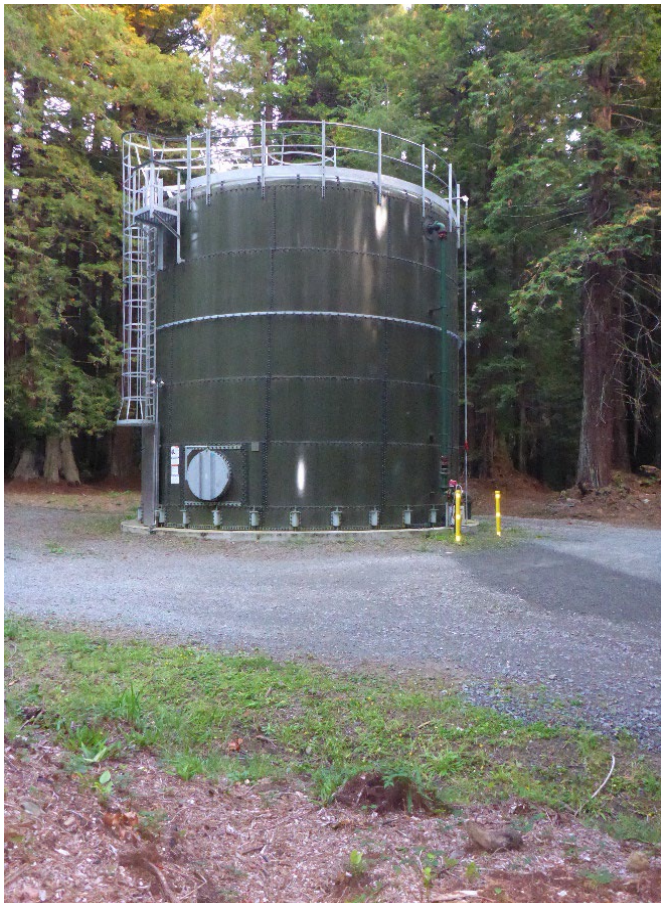
Existing Glass-Fused Bolted Steel Tank
