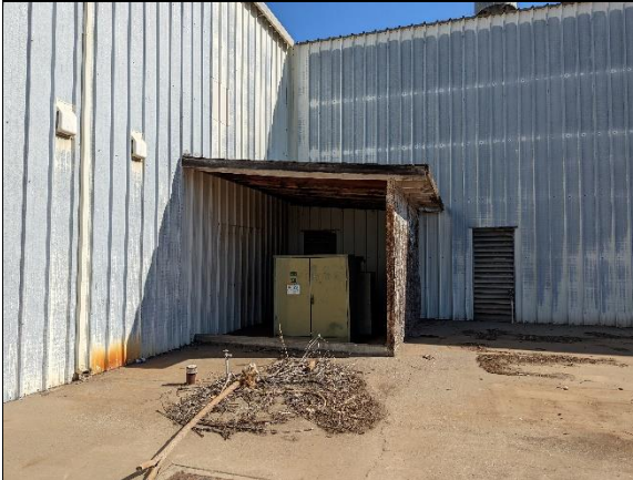
Photograph 13. View of pad-mounted transformer located on the south wall of the storage warehouse.
