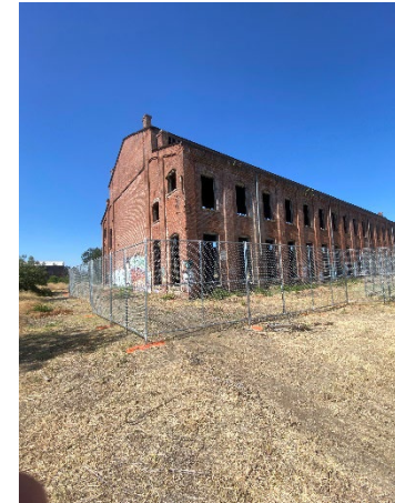
Photograph 12: Vacant building in western portion of BYSP Area.
