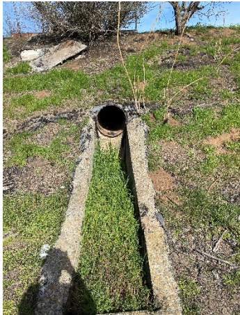
Photograph 10: Culver within detention basin, looking east.
