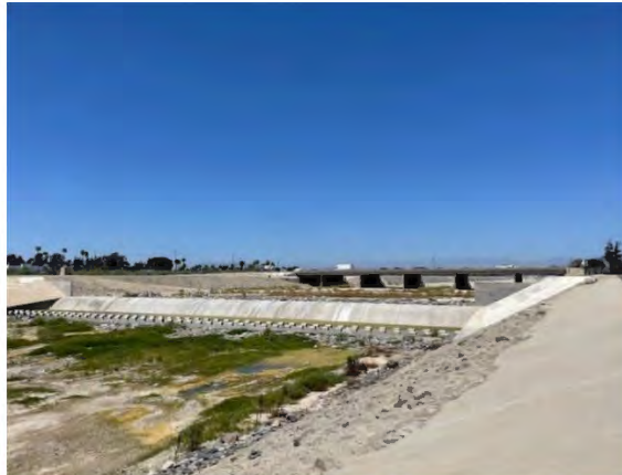
Photograph 41: East side of project site from pedestrian trail, facing northwest.
