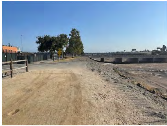
Photograph 2: Project site from Orangewood Avenue, facing north.
