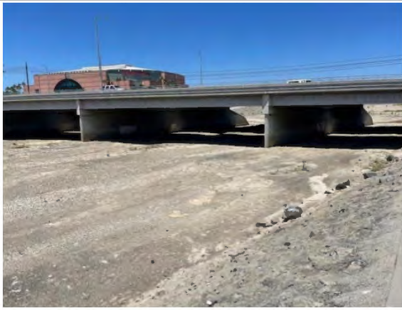
Photograph 37: East side of project site from pedestrian trail, facing northwest.
