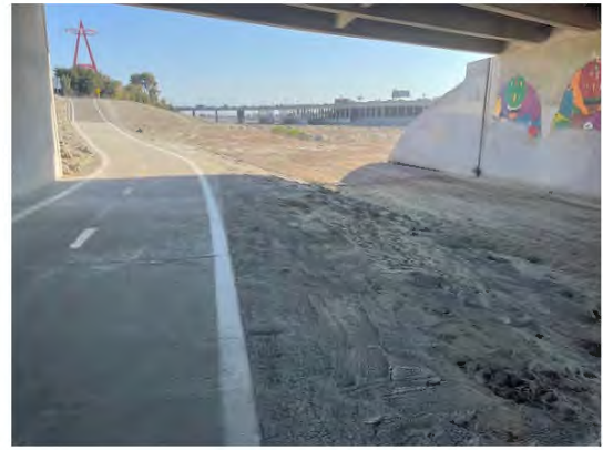
Photograph 3: Project site between Orangewood Avenue and Katella Avenue, facing north.
