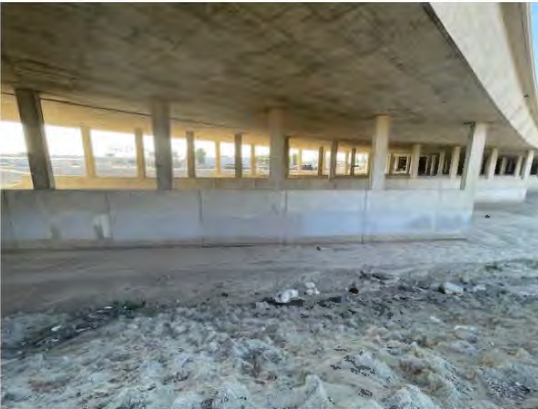
Photograph 4: Katella Avenue underpass, facing east.
