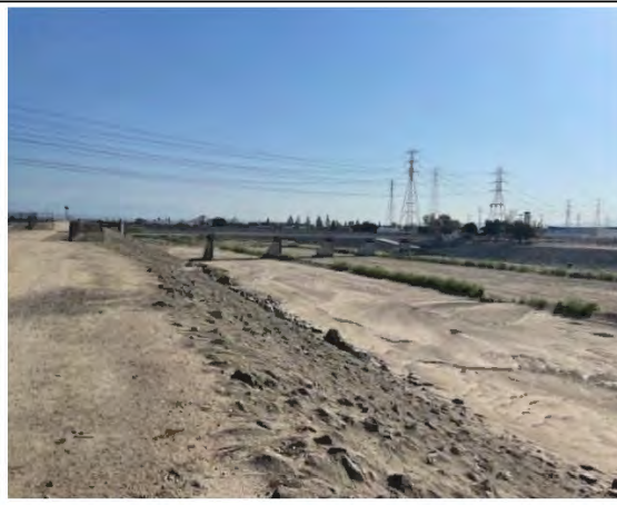
Photograph 20: Project site between Katella Avenue and East Ball Road, facing northeast.
