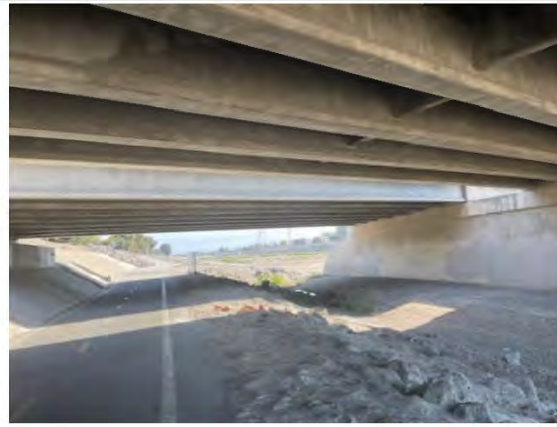
Photograph 11: Katella Avenue underpass, facing north.
