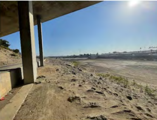
Photograph 5: Katella Avenue underpass, typical ground visibility, facing north.
