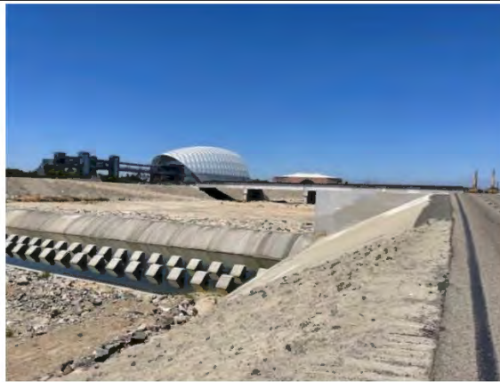
Photograph 35: East side of project site, facing northwest.
