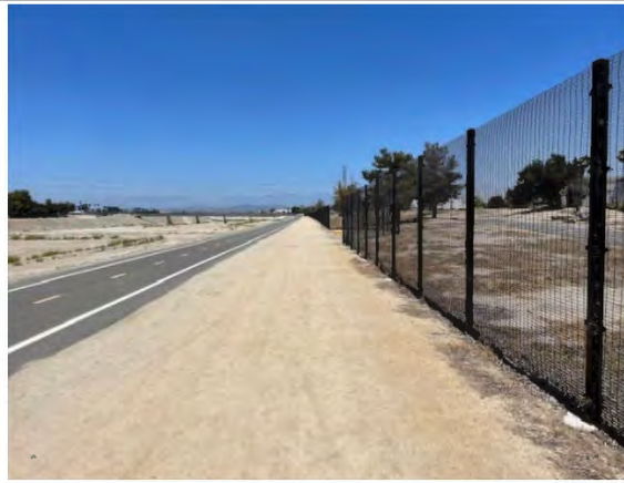
Photograph 38: East side of project site from pedestrian trail, facing north.
