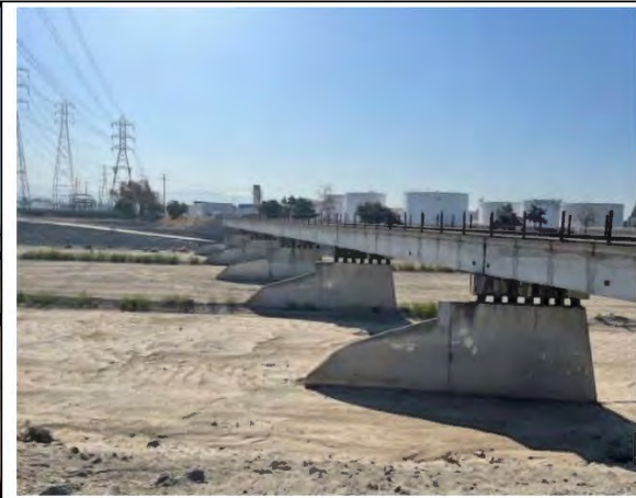
Photograph 21: North portion of railroad tracks, facing east.
