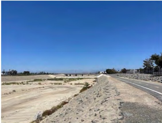
Photograph 40: East side of project site from pedestrian trail, facing north.
