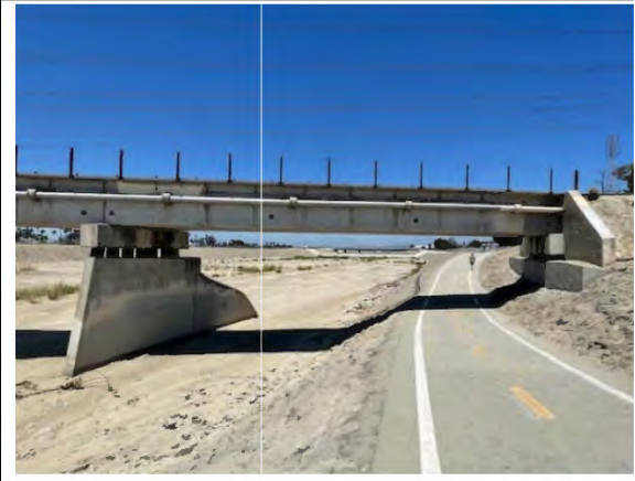
Photograph 39: East side of project site from pedestrian trail, facing north.
