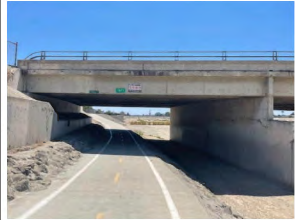
Photograph 42: East side of project site, facing south towards Taft Street.
