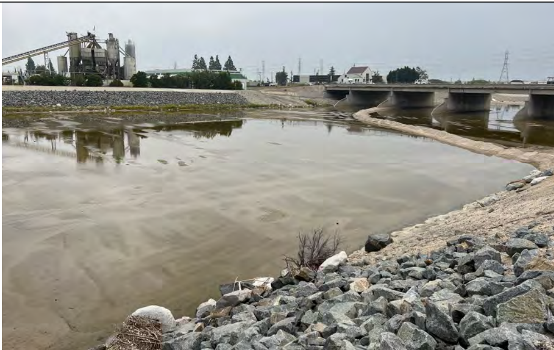
Photograph 2: Location: 33.817237 N, -117.870209 W) Southeast-facing view of the northern extent of the Santa Ana River in the survey area. This photograph shows the flowing water through the center of the concrete- and riprap-lined channel. Also shown in the right-hand side background of the photograph is the consolidated deposited sediments in the center of the channel.
