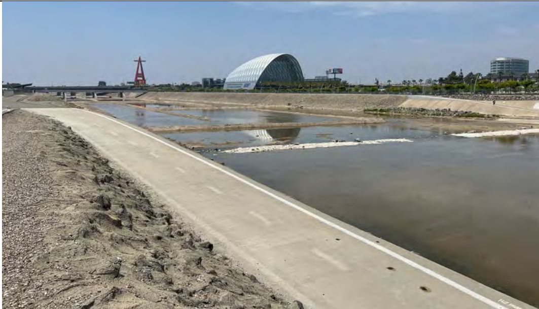
Photograph 6: (Location: 33.805756 N, -117.874260 W) Southwest-facing view of the Santa Ana River in the south-central portion of the survey area. Surface water and deposited saturated soils are visible in the bottom of the concrete- and riprap-lined channel.
