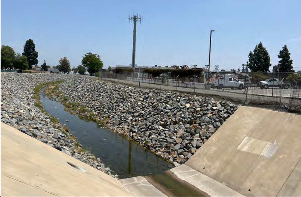
Photograph 9: (Location: 33.803901 N, -117.874955 W) Northeast-facing view of Collin's Channel showing where sampling point NW-2-1 was collected to document the presence of OHWM indicators. This photograph shows the riprap and concrete lining the channel. The sparse weeds and grasses growing through the riprap and surface water in the center of the channel are also shown in the center and background of the photograph.
