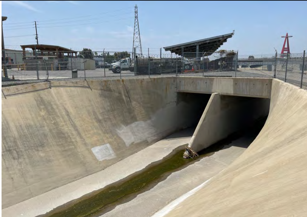
Photograph 10: (Location: 33.803901 N, -117.874955 W) Southwest-facing view of Collin's Channel showing where sampling point NW-2-2 was collected to document the presence of OHWM indicators. This photograph shows the concrete-lined channel, surface water flowing through the center, and the box culvert through which Collin's Channel connects to the Santa Ana River channel.
