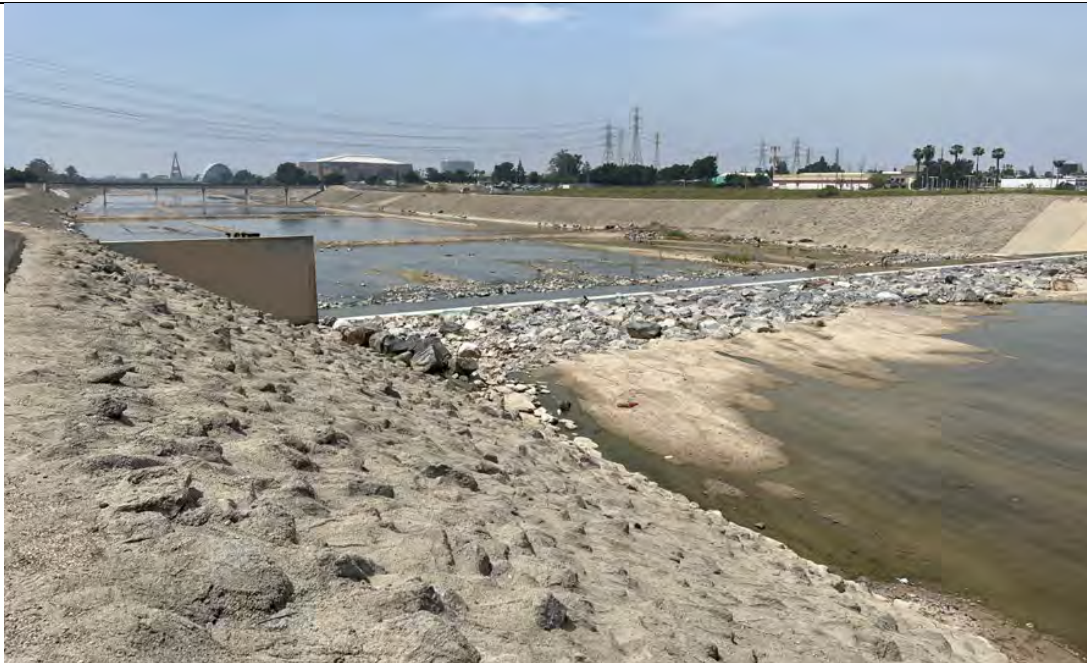
Photograph 4: (Location: 33.815586 N, -117.869401 W) Southwest-facing view of the Santa Ana River downstream of where sampling point NW-1-1 was collected. A concrete spillway and riprap that occur across the center of the concrete-lined channel are visible in the center of the photograph.
