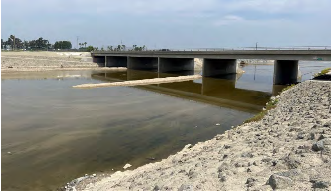
Photograph 3: (Location: 33.815586 N, -117.869401 W) Northwest-facing view of the Santa Ana River in the northwestern portion of the survey area where sampling point NW-1-1 was collected. Flowing water and deposited soils in the bottom of the channel are visible in the center of the photograph.
