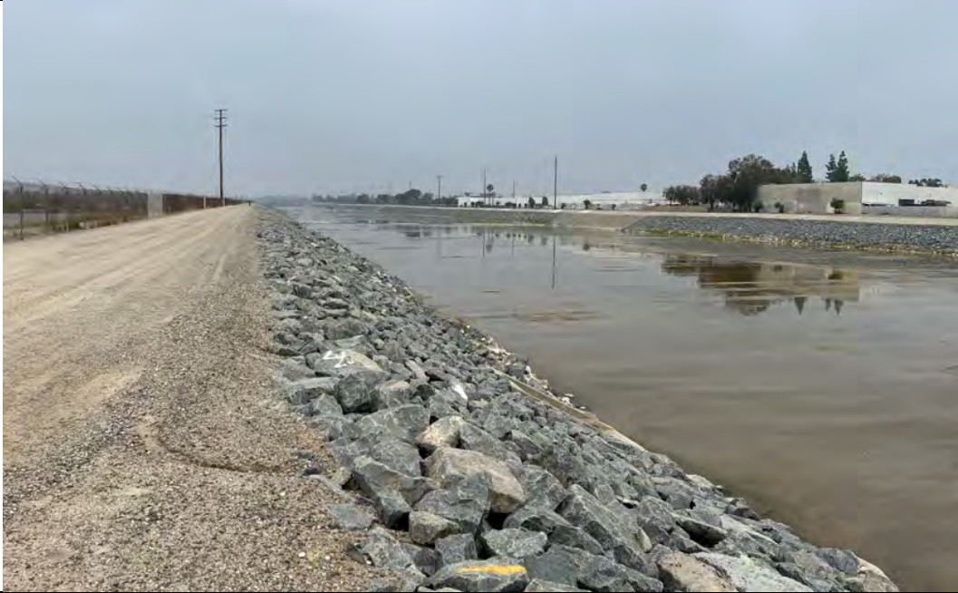
Photograph 1: (Location: 33.817237 N, -117.870209 W) Northeast-facing view of the northern extent of the Santa Ana River where the concrete- and riprap-lined channel enters the northeastern portion of the survey area. This photograph shows the concrete-lined channel and riprap-lined banks of the river. Surface water is also visible in the bottom of the river channel.
