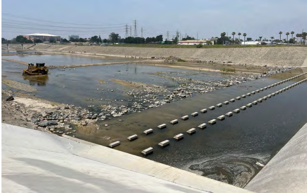
Photograph 5: (Location: 33.815202 N, -117.869595 W) Southwest-facing view of the Santa Ana River south of a spillway in the northern portion of the survey area. This photograph shows the heavy equipment being used to move deposited sediment in the bottom of the concrete- and riprap-lined channel.
