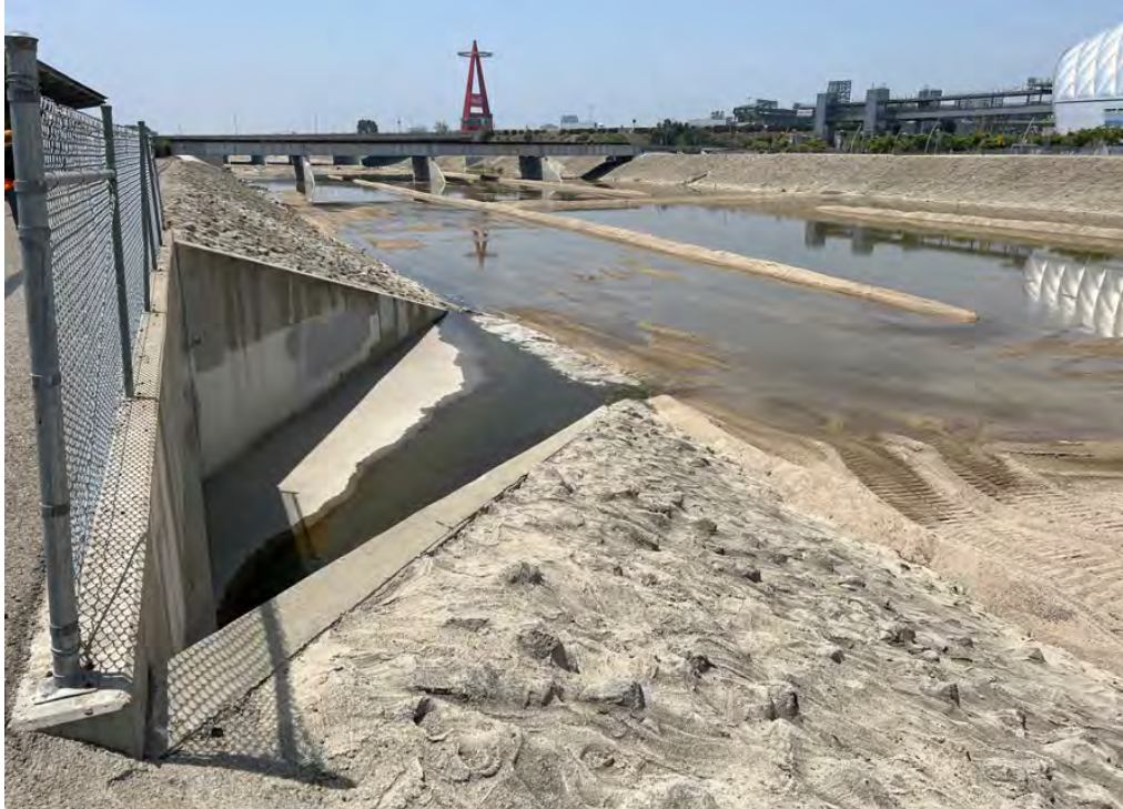
Photograph 11: (Location: 33.803491 N, -117.875346 W) This photograph shows where Collin's Channel connects to the Santa Ana River channel through a concrete box culvert. The surface water flowing from Collin's Channel into the Santa Ana River channel is shown in the center of the photograph.
