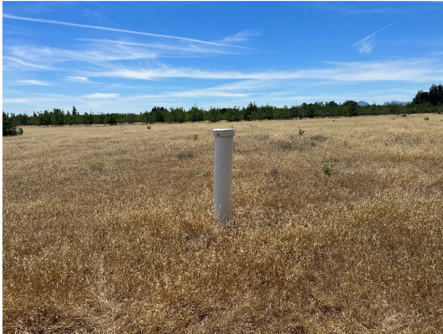
Photograph 9, view facing south: A 10-inch diameter, 4 ft tall vertical, capped PVC pipe.
