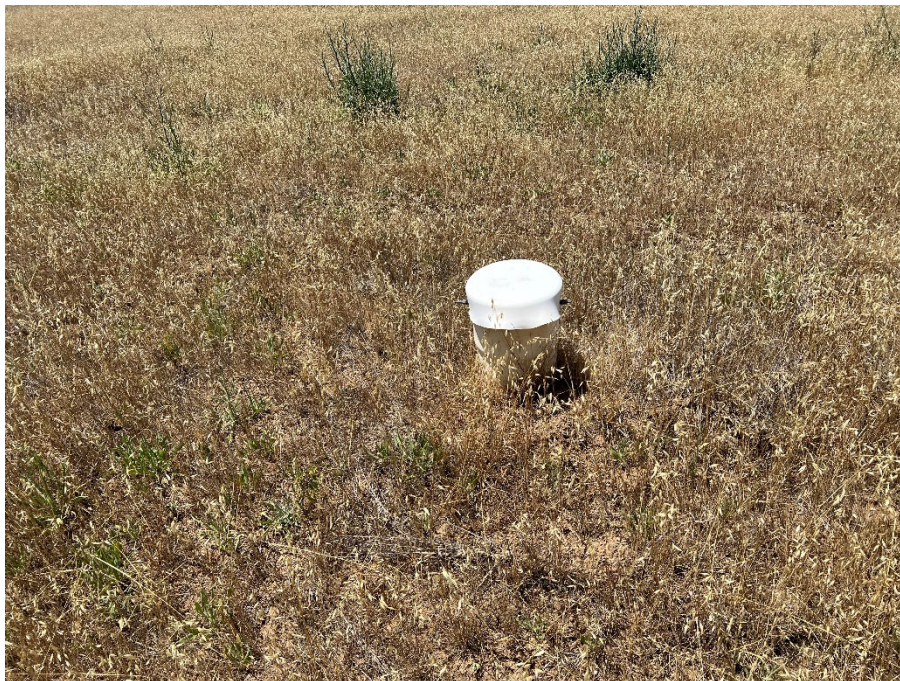
Photograph 13, view facing northwest: Example of 10-inch diameter capped PVC vertical pipes.
