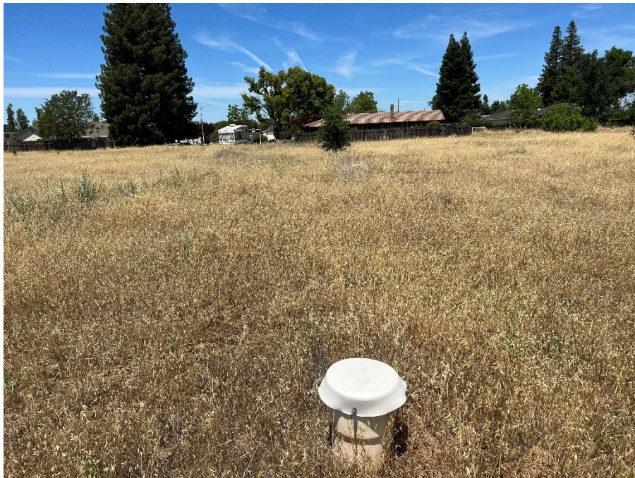
Photograph 14, view facing north: 10-inch capped PVC vertical pipe.
