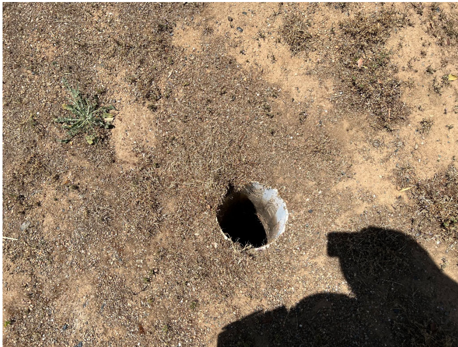
Photograph 11, view facing down: 10-inch PVC pipe flush with ground surface located at the north edge of Subject Property. Depth and purpose undetermined.
