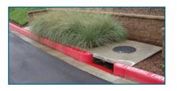
biological process working to break down and remove non-point source pollutants. The flow rate is controlled in the MWS Linear, giving the plants more contact time so that pollutants are more successfully decomposed, volatilized, and incorporated into the biomass of the Modular Wetlands'® micro/macro flora and fauna.
