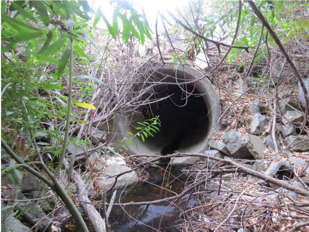
**Photograph 19:** Main culvert that conveys flows into Drainage 1 on the southeast corner of the site.
