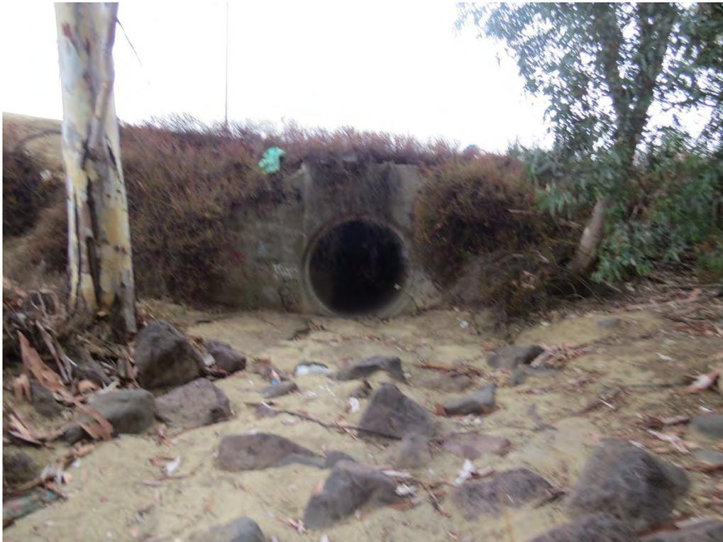
**Photograph 26:** Looking at the culvert at the western end of Drainage 1 that receives water flows from Drainage 1 and conveys under Murrieta Hot Springs Road.
