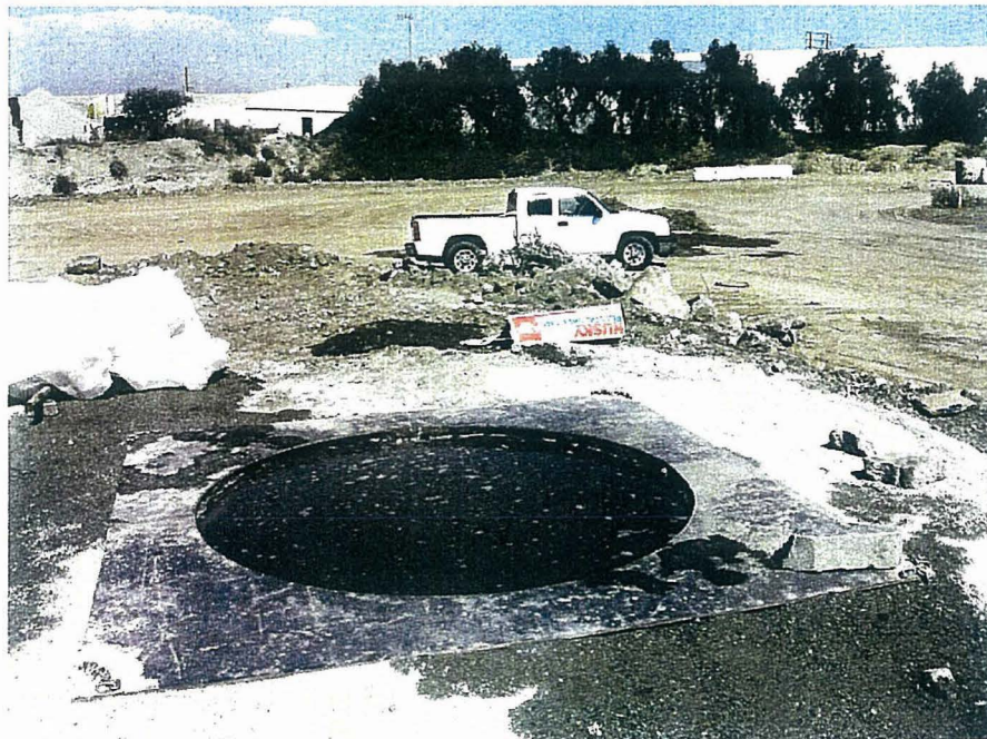
Ring Density Pits in Properly Compacted Debris Fill
