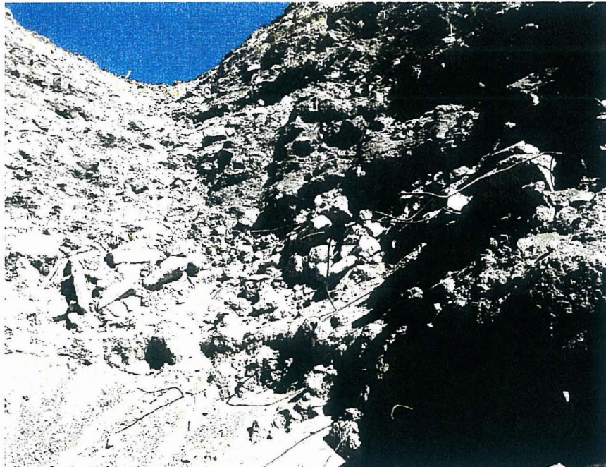
Test Pit Walls
