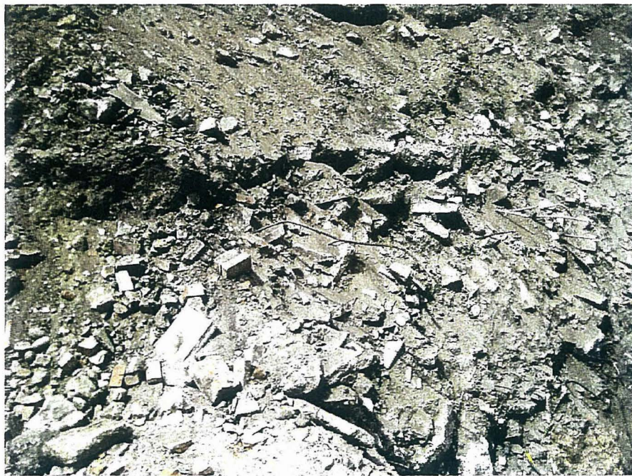
Test Pit Walls
