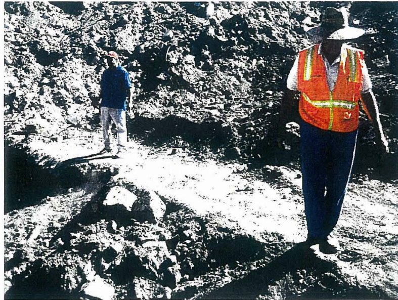
East Trench Concrete Footing at Depth of Approximately 20 Feet Below Ground Surface
