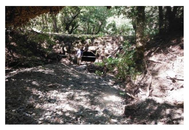
Figure 28. Sediment accumulation, North Fork Mark West Creek above culvert at the St. Helena Road crossing (May 2013).
