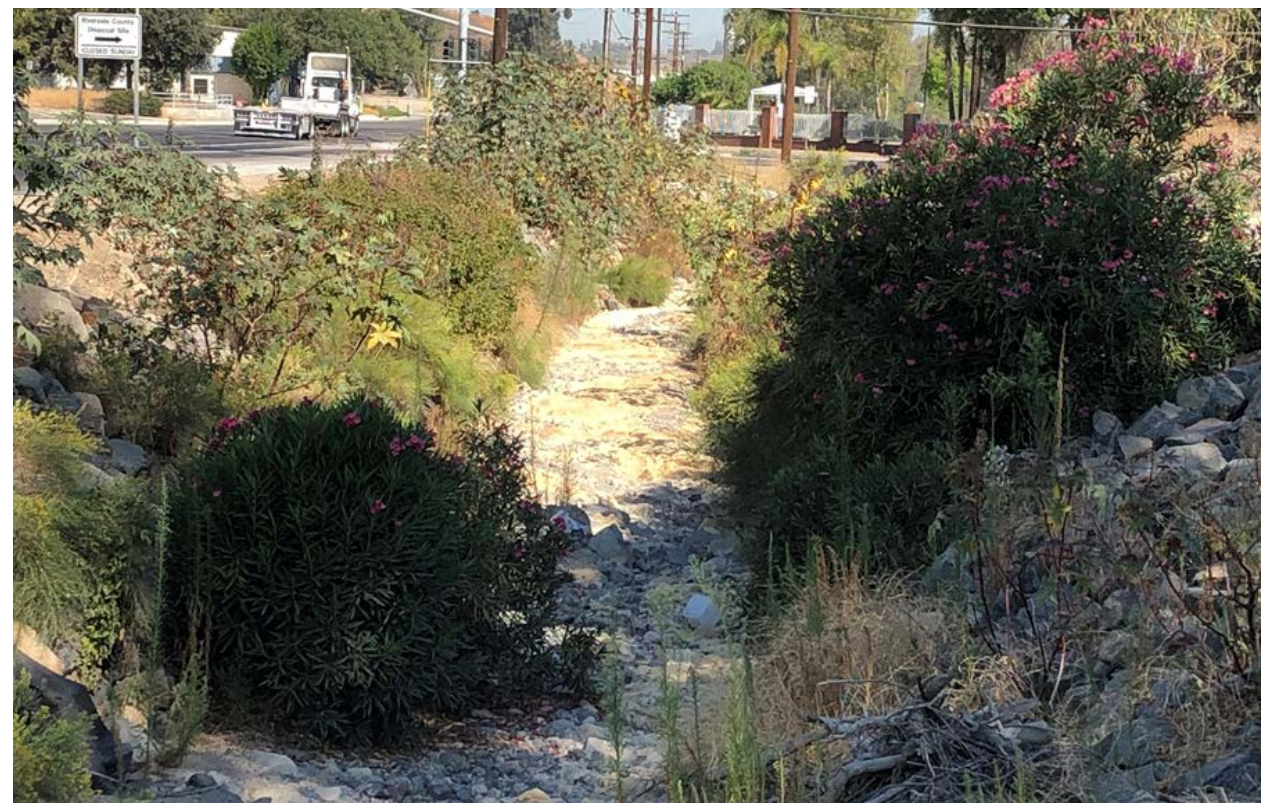
Photograph 2: Coldwater Creek looking downstream near northern project boundary showing unvegetated channel and banks with upland vegetation.
