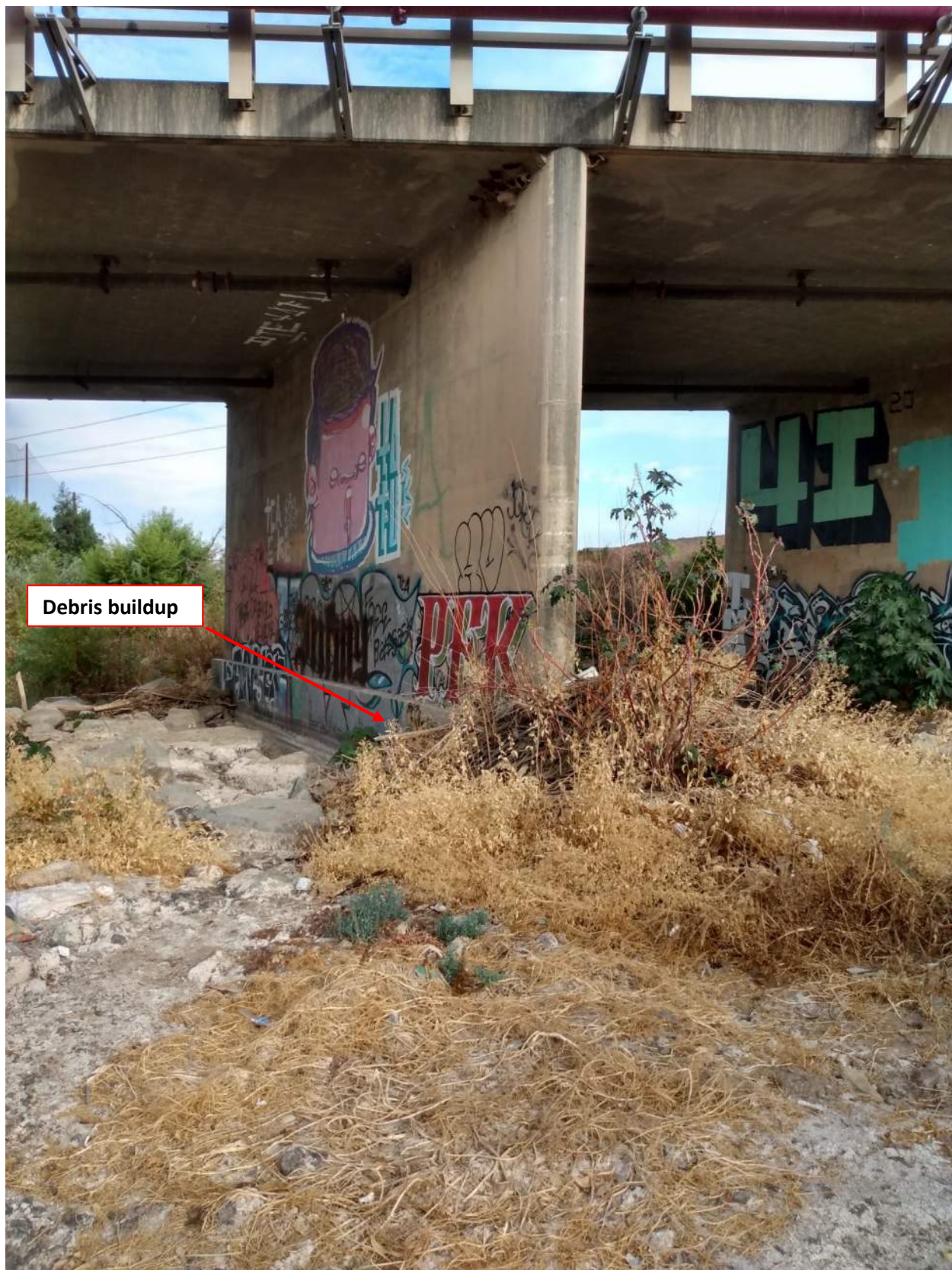
Photo 9: Pier 4 photo taken on upstream side of bridge looking north
