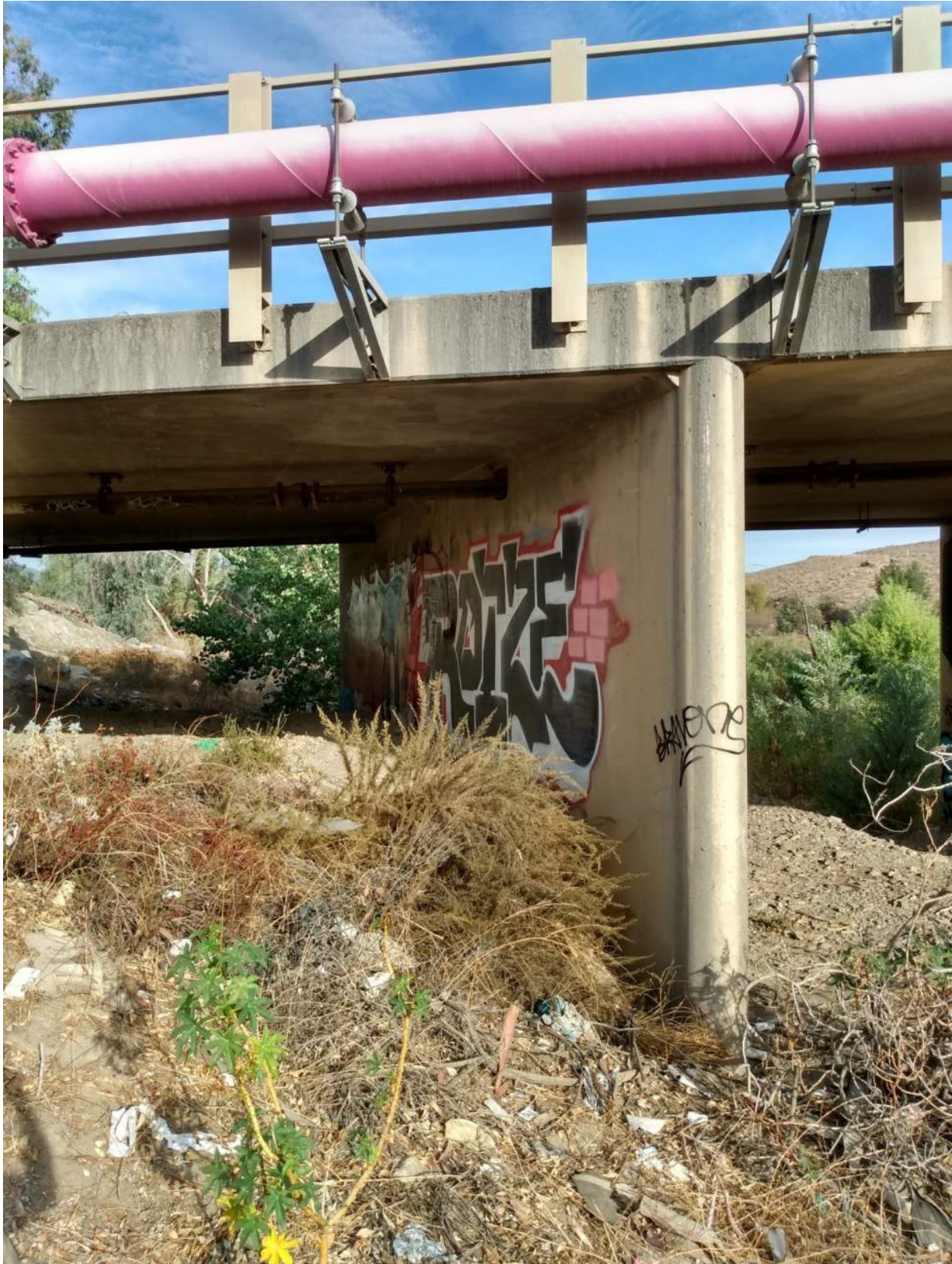
Photo 3: Pier 2 photo taken on upstream side of bridge looking north
