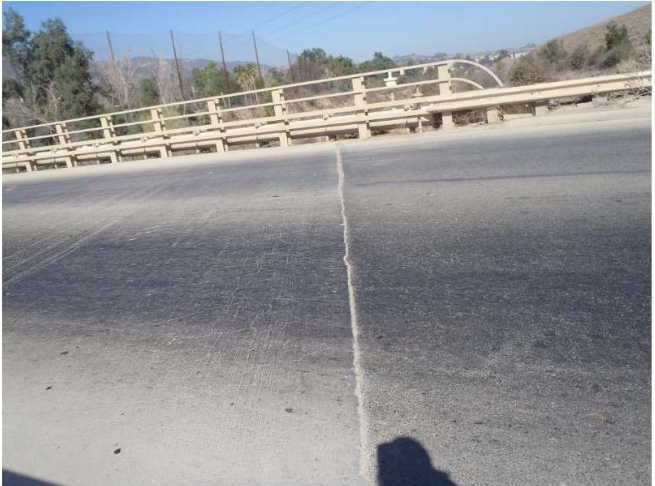
Photo No. 1 JOINT CONDITION ABOVE NORTHERN ABUTMENT (ABUTMENT 6)
