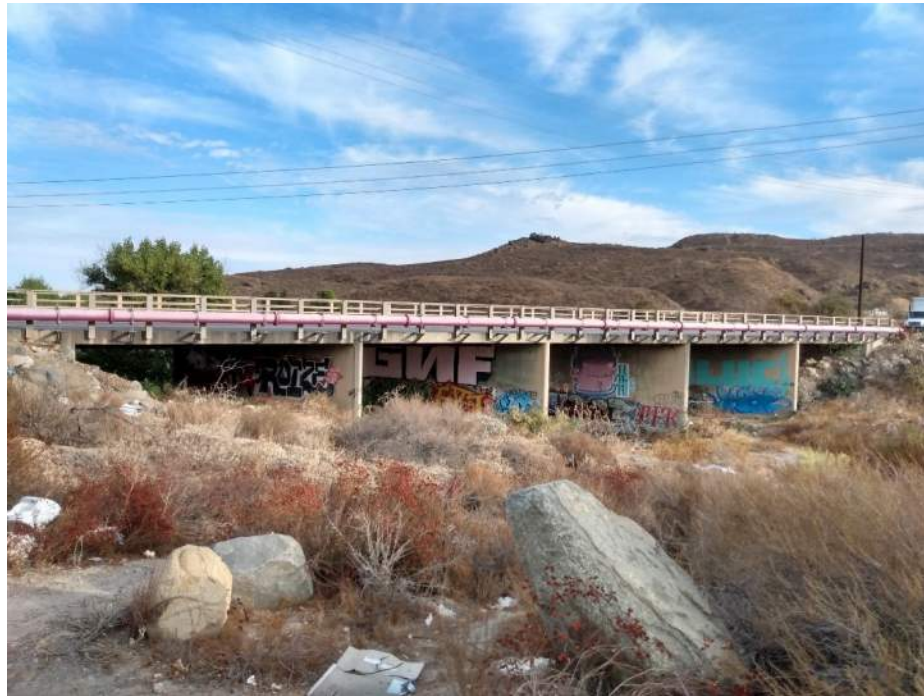
Photo 1: Elevation View of Bridge (Looking North)
