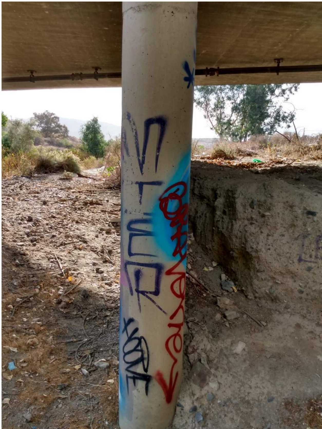
Photo 5: Pier 2 photo taken on downstream side of bridge looking south
