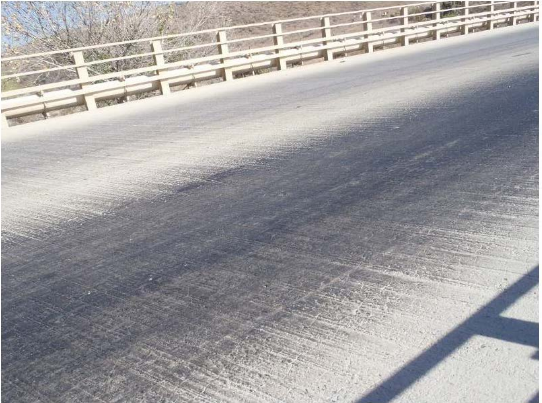
Photo No. 1 TYPICAL DECK SURFACE CONDITION
