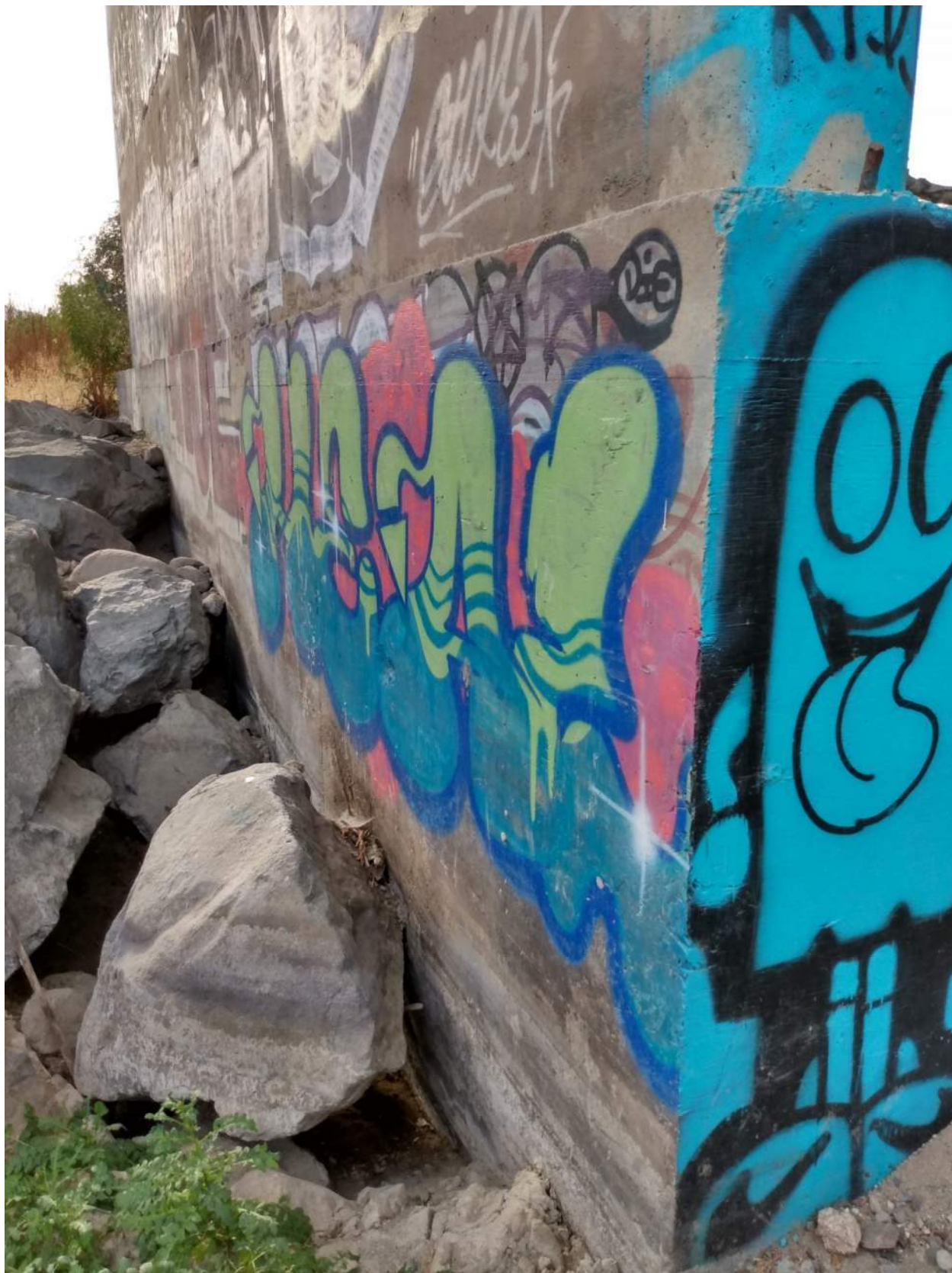
Photo 7: Pier 3 photo taken on downstream side of bridge looking south
