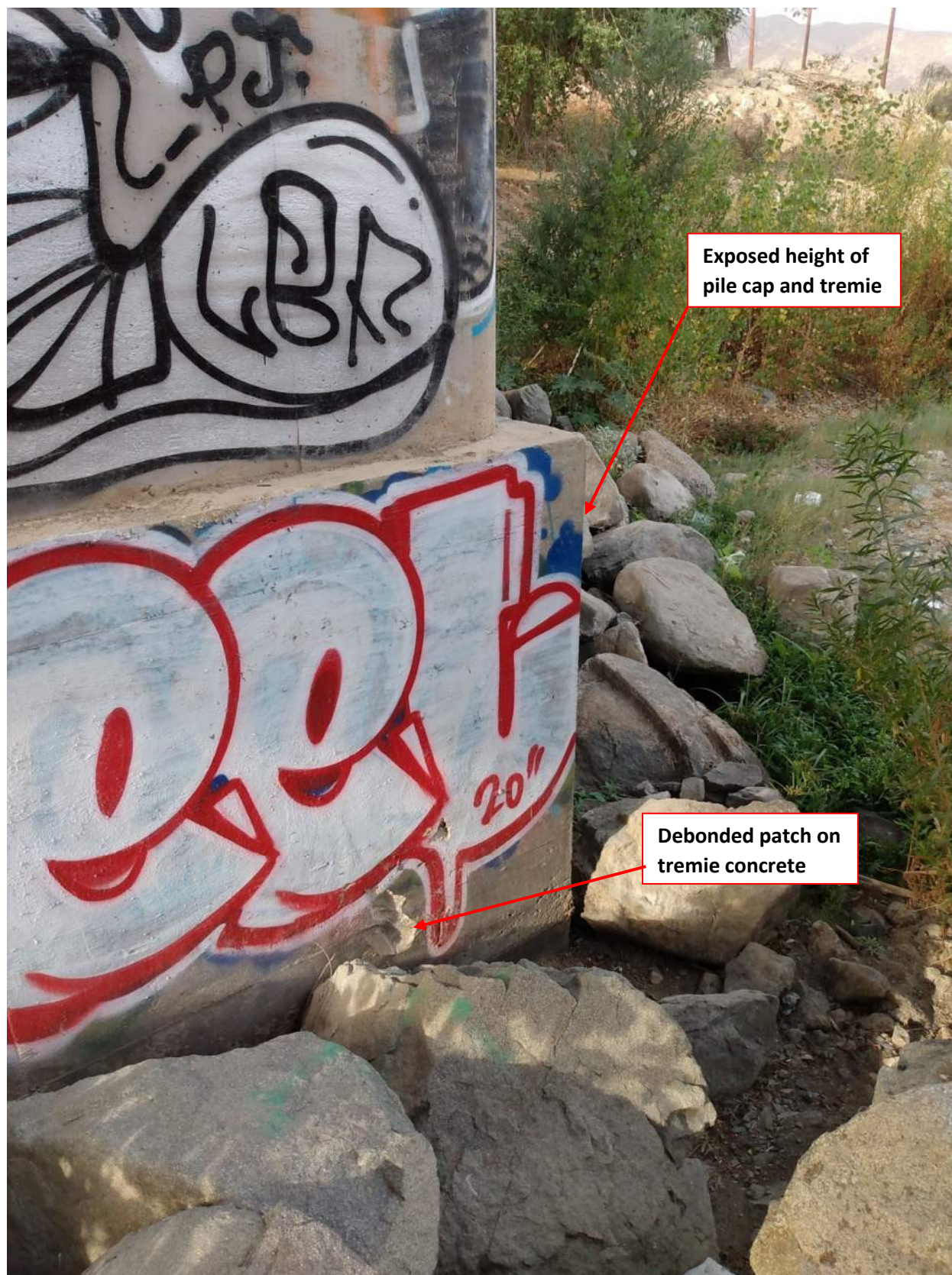
Photo 11: Pier 4 photo taken on downstream side of bridge looking west
