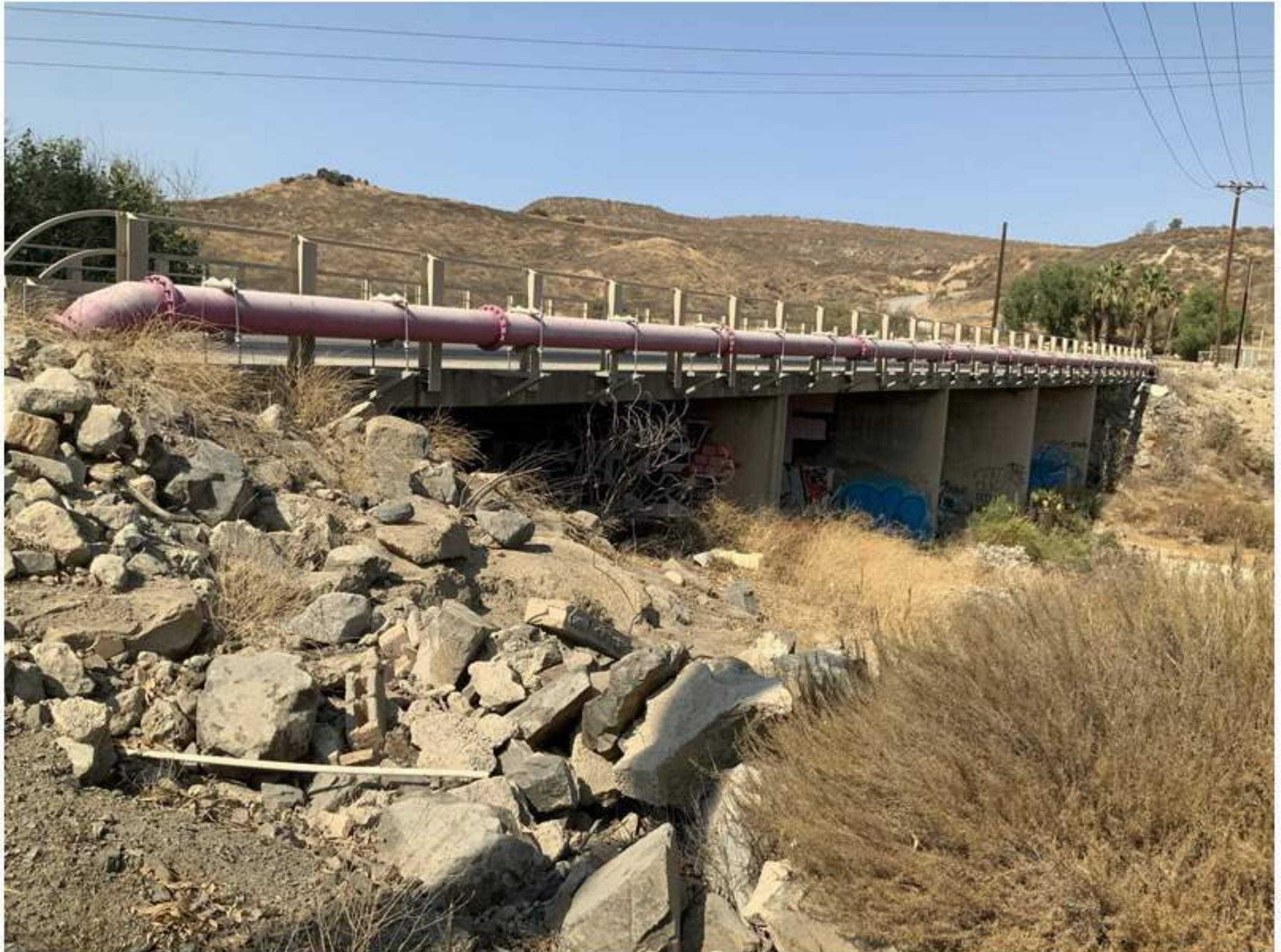
Photo No. 102 Elevation View Looking North
