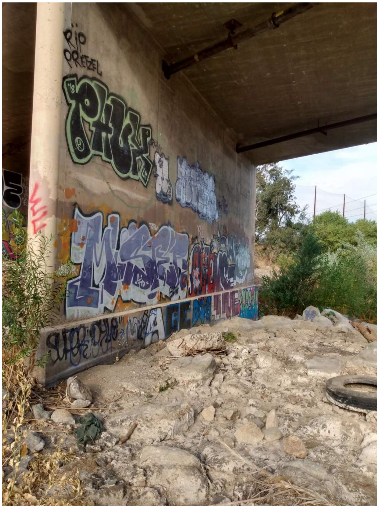
Photo 8: Pier 3 photo taken on upstream side of bridge looking west
