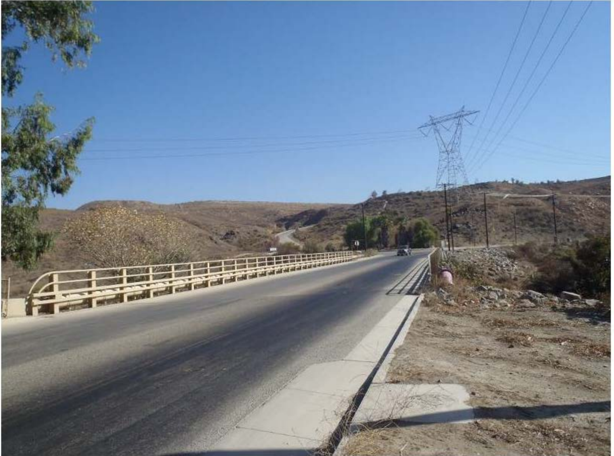
Photo No. 1 ROADWAY VIEW LOOKING NORTHEAST
