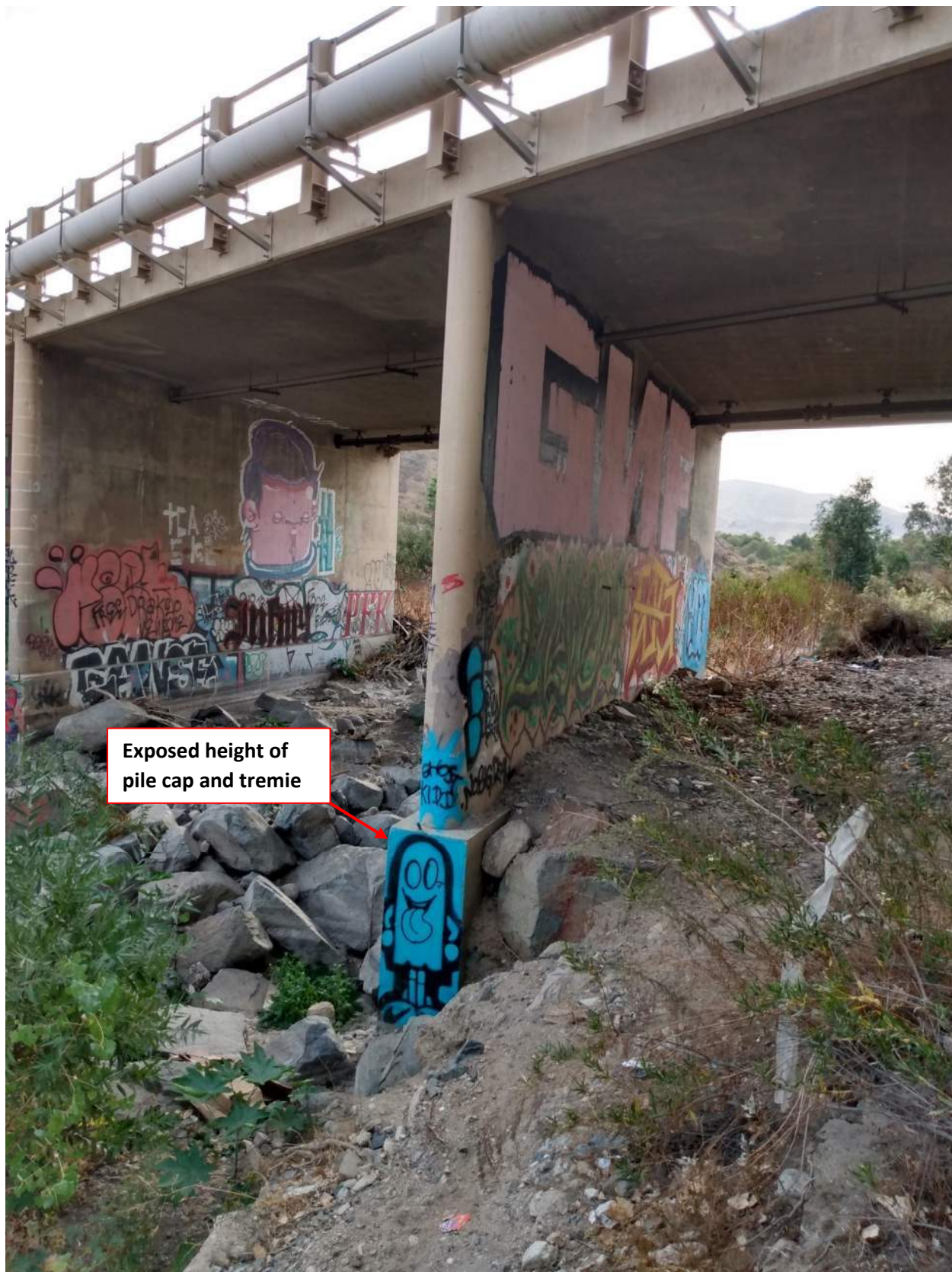
Photo 6: Pier 3 photo taken on downstream side of bridge looking south
