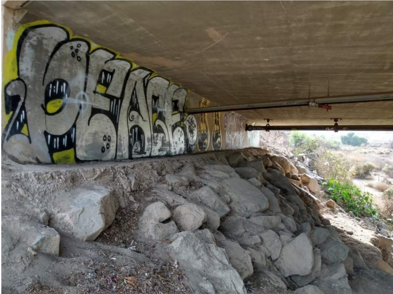
Photo 14: Abutment 6 photo taken on downstream side of bridge looking east
