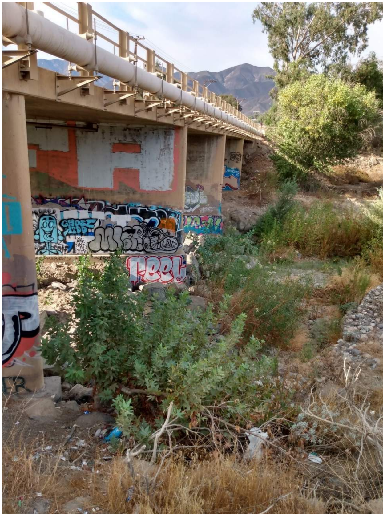
Photo 15: Elevation view taken on downstream side of bridge looking west
