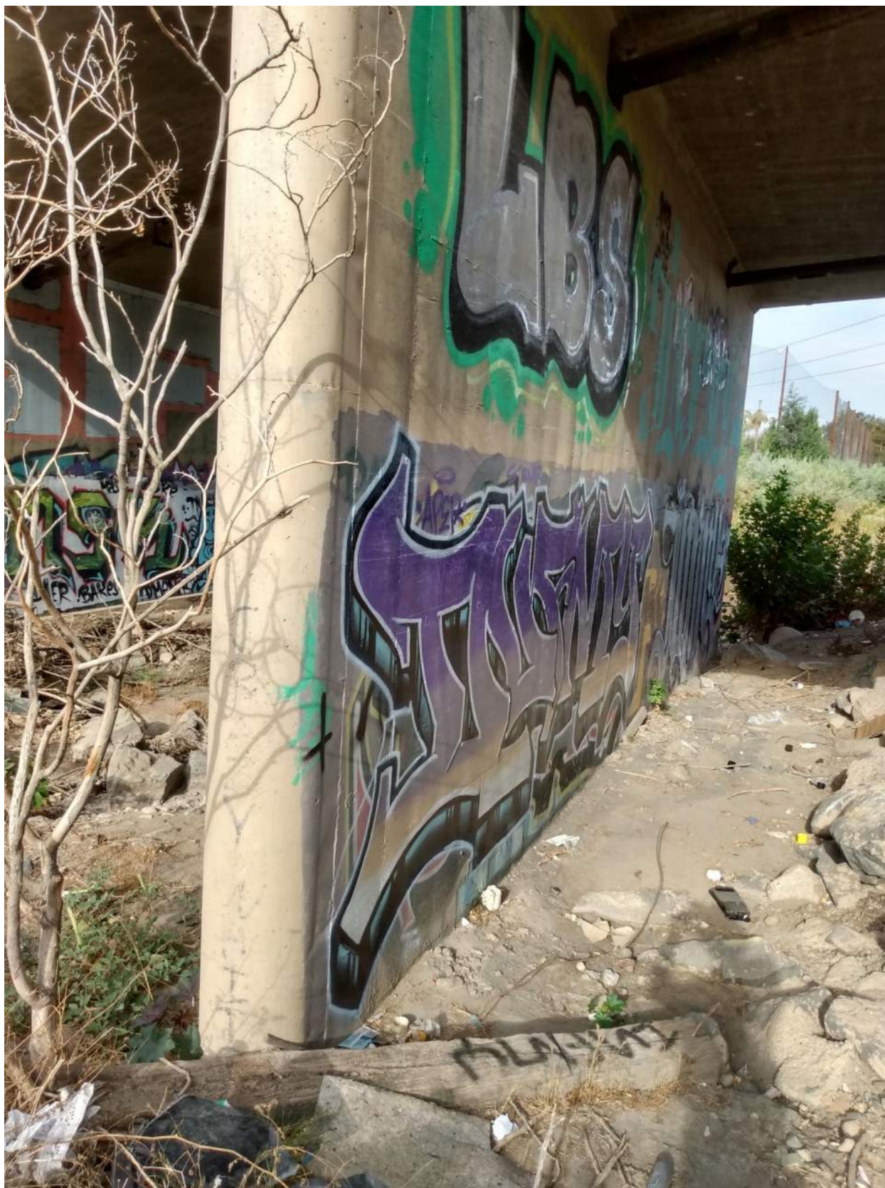
Photo 13: Pier 5 photo taken on upstream side of bridge looking west
