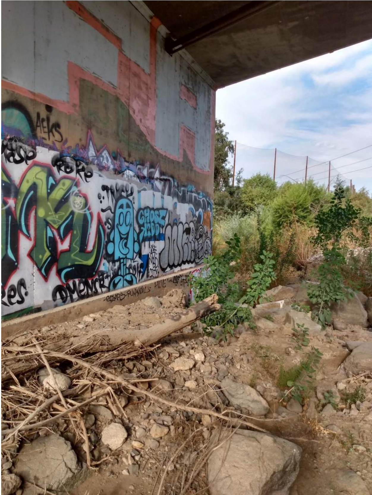
Photo 10: Pier 4 photo taken on upstream side of bridge looking west
