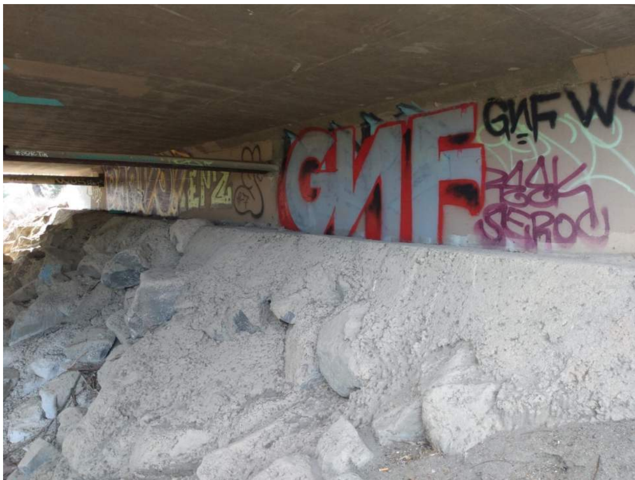
Photo 4: Abutment 1 photo taken on downstream side of bridge looking west
