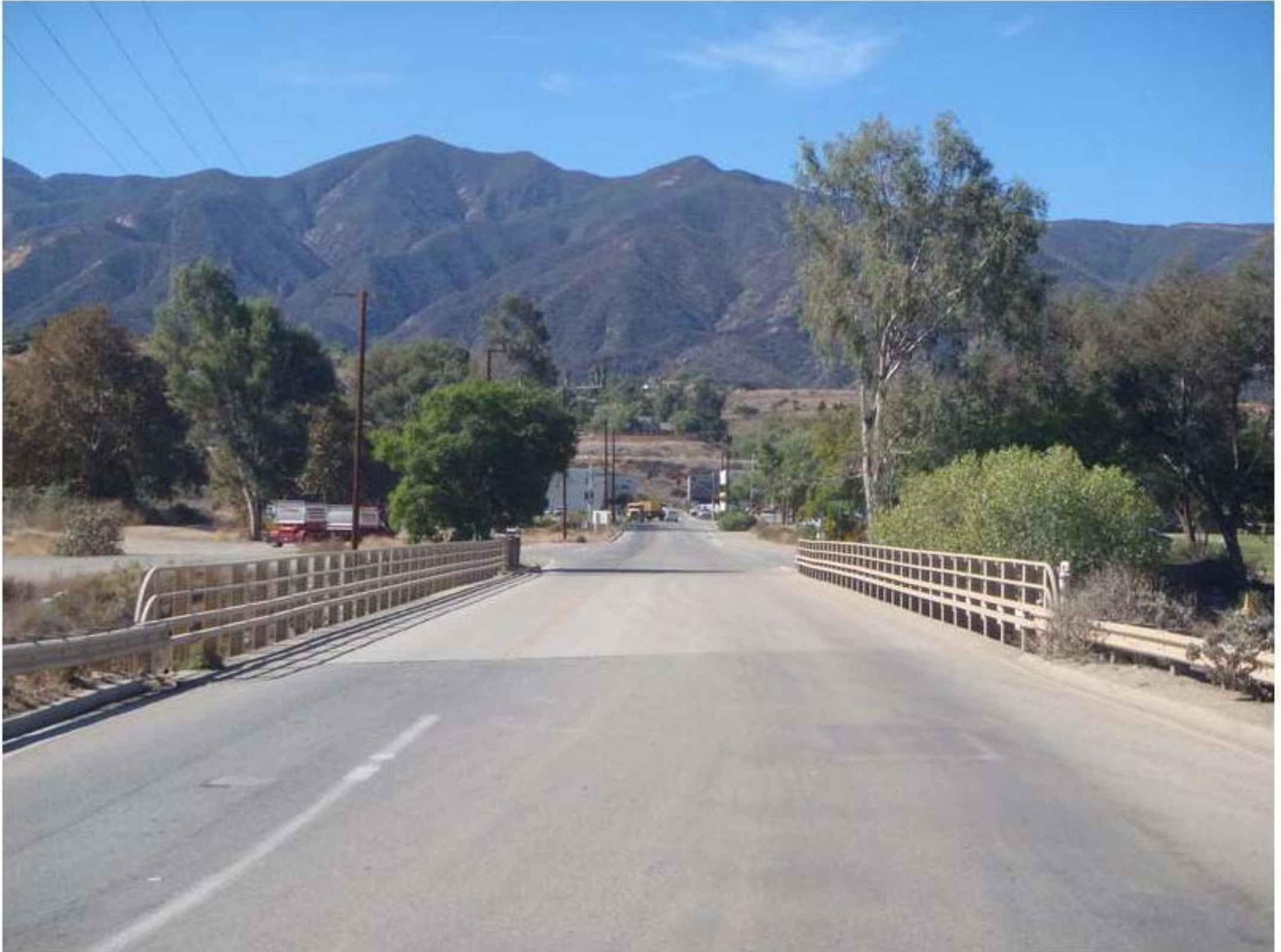
Photo No. 1 Roadway View Looking West
