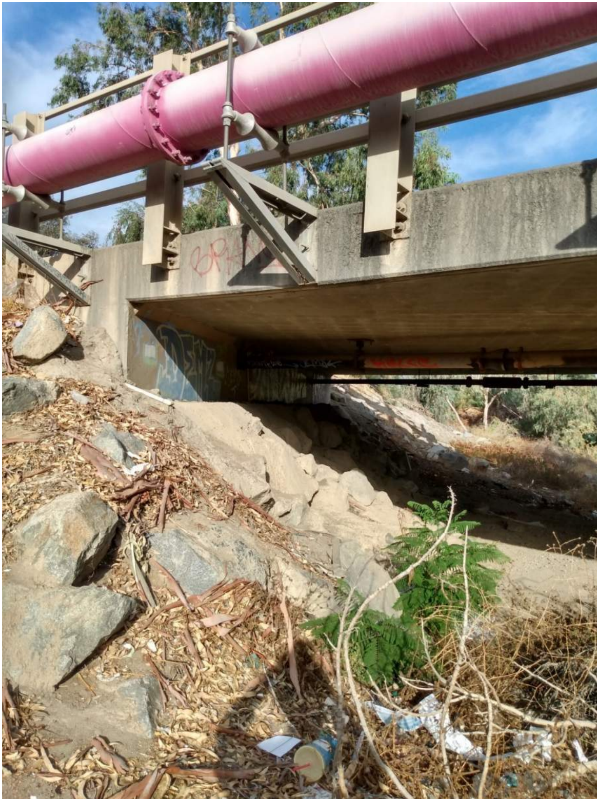
Photo 2: Abutment 1 photo taken on upstream side of bridge looking west
