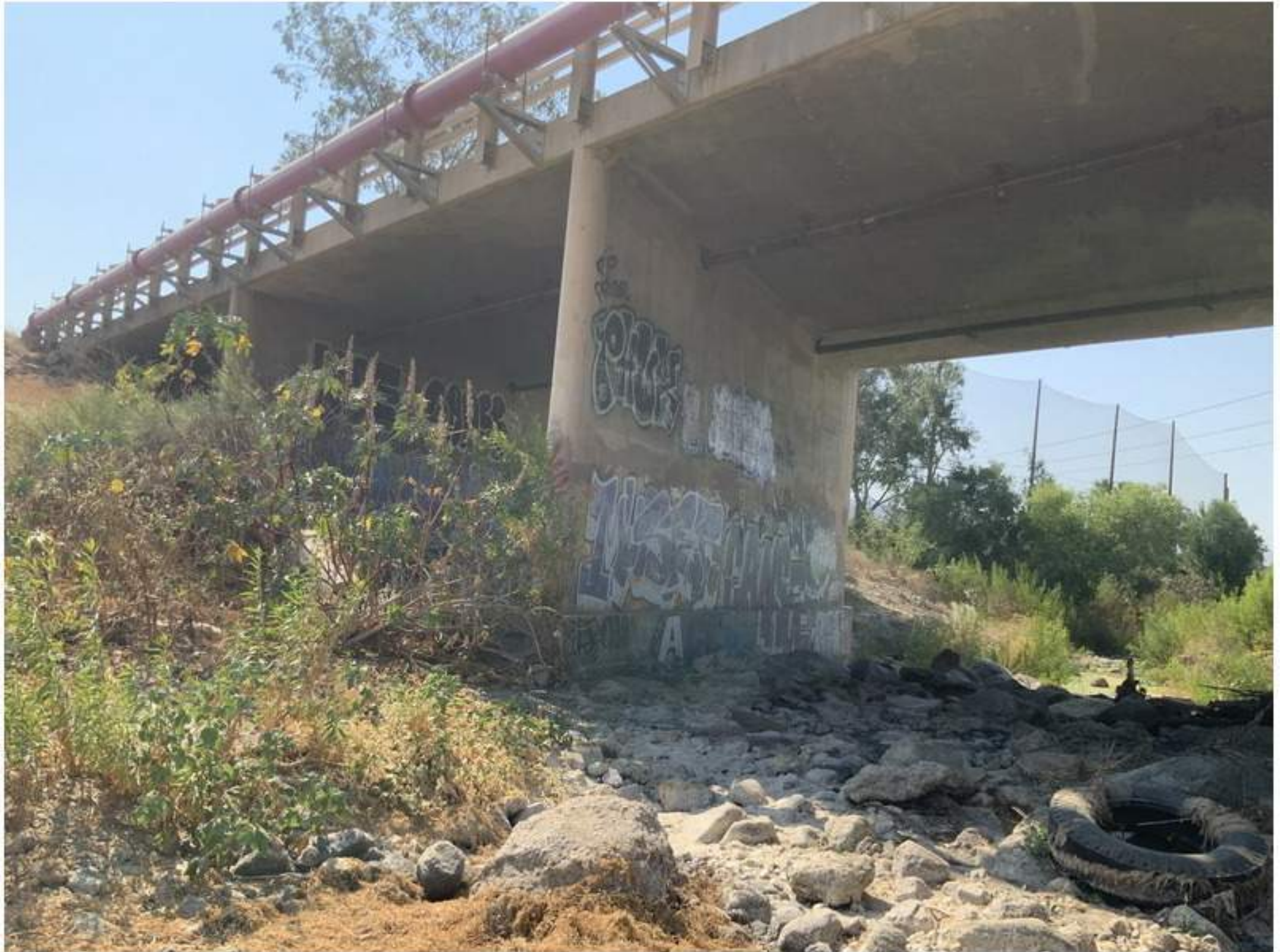
Photo No. 105 Exposed Pier Wall Footings
