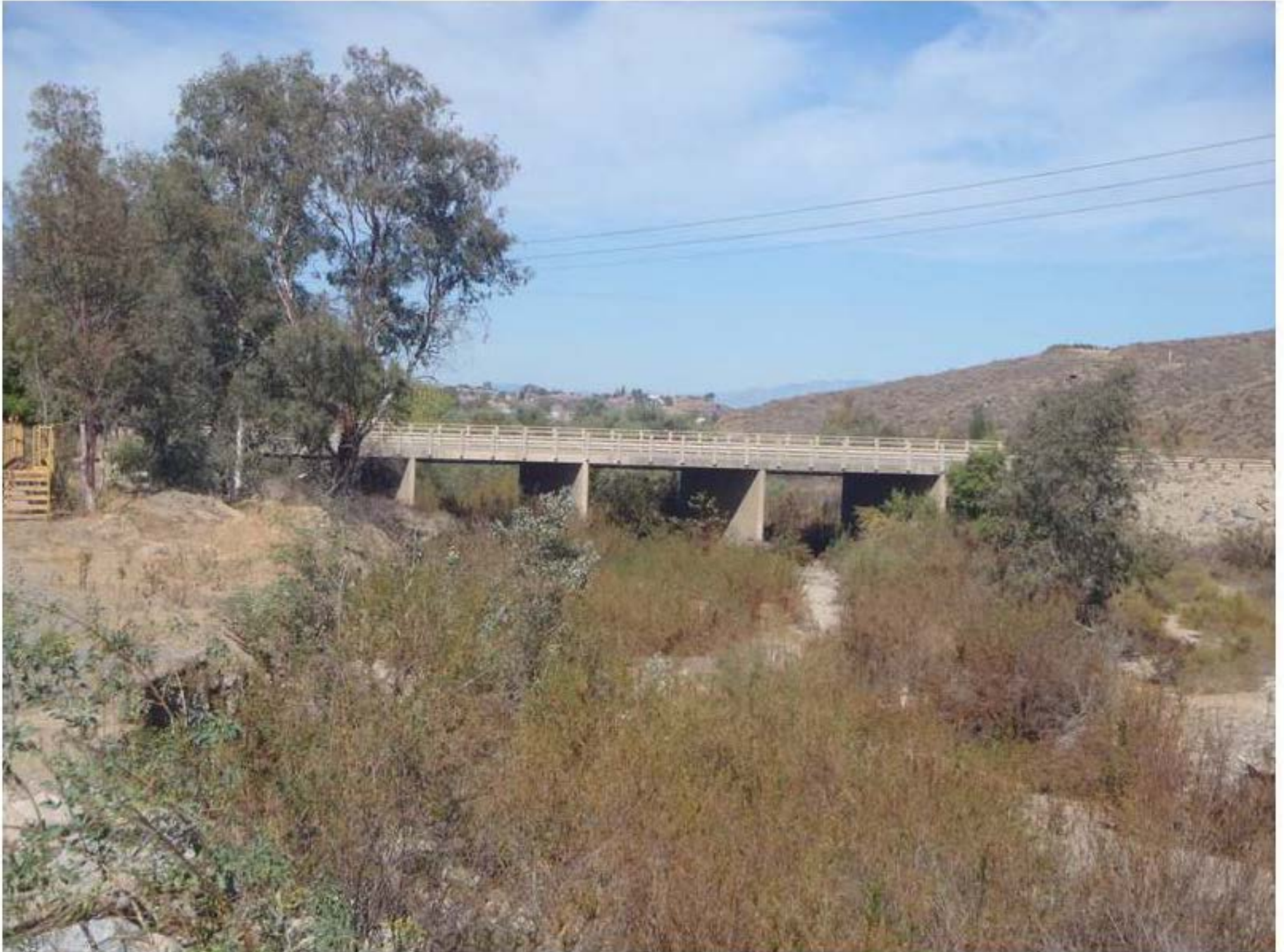
Photo No. 1 Elevation View Looking North
