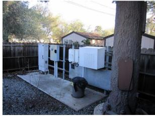
Photograph 4. Cellular telephone equipment enclosure.
