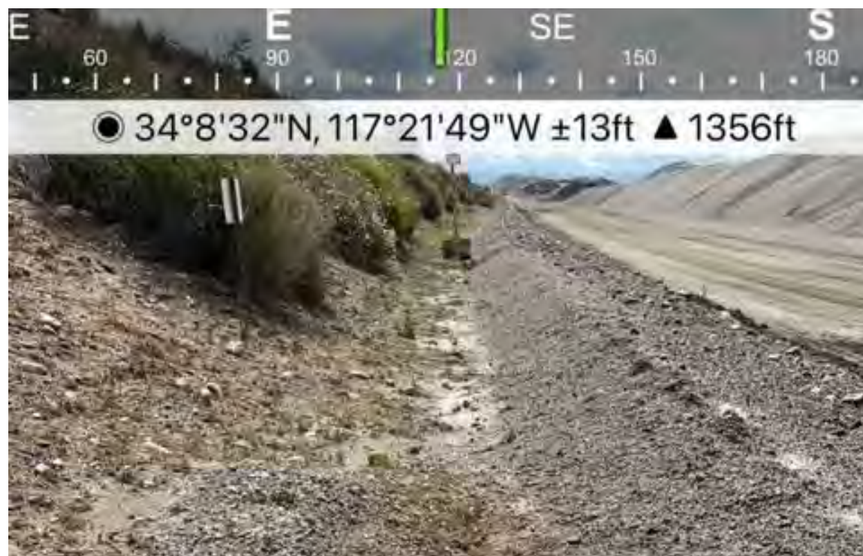
Photograph 5: View of the western toe of the eastern levee showing fine surface materials, which was determined not to be suitable for SBKR.
