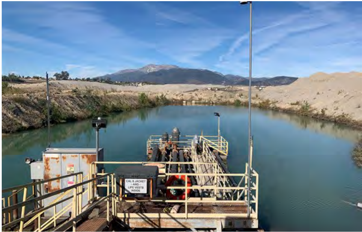
Photograph 2: Representative photo of Settling Basin B within the Project site. Settling Basin B includes three interconnected basins.
