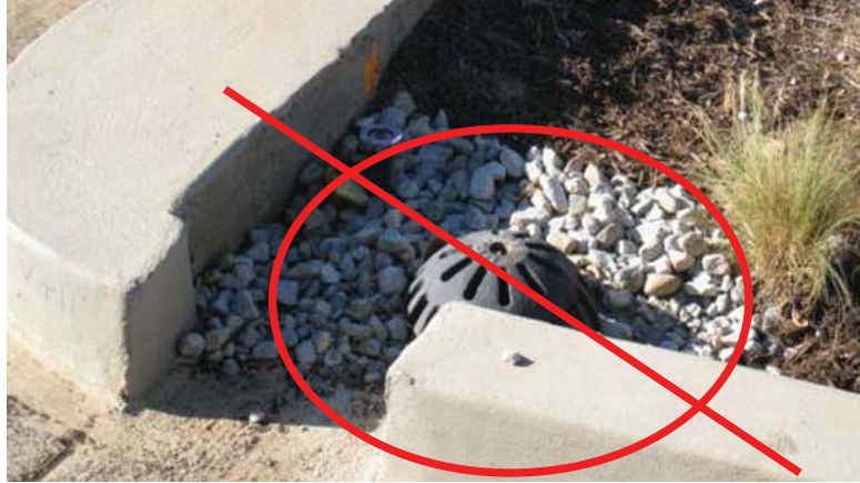
Figure 6: Incorrect Placement of an Overflow Inlet.
