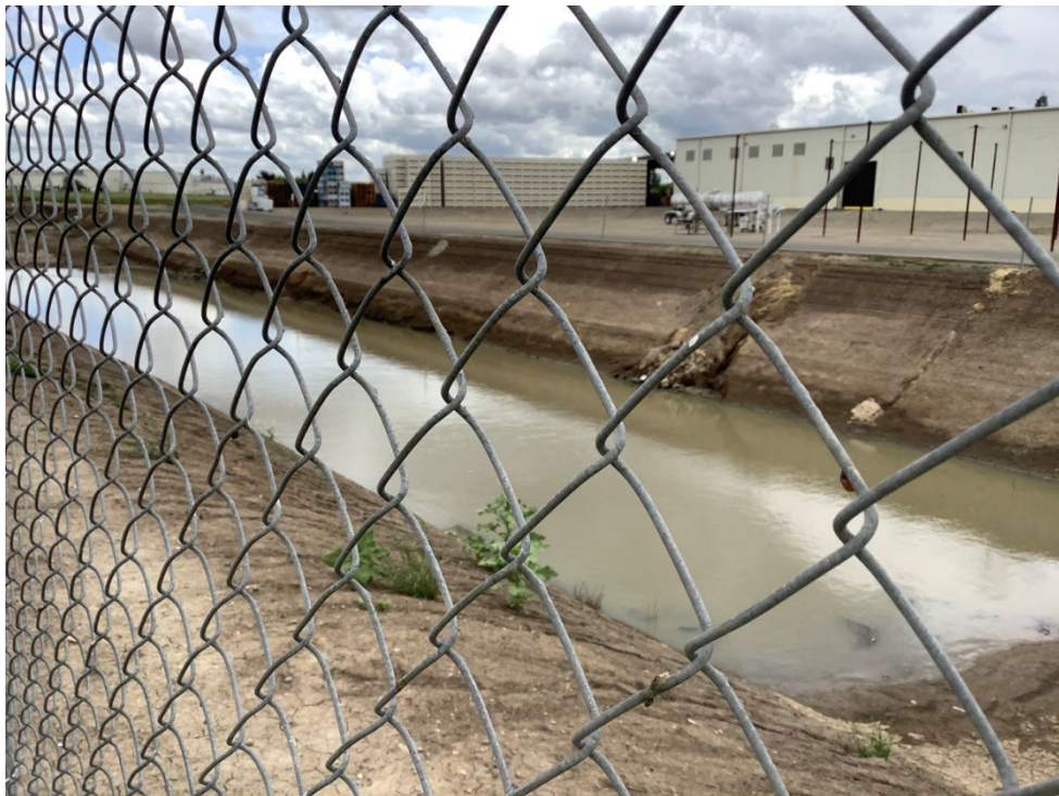
Photo 10. Upland detention basin south of Fahrens Creek, looking east. May 2, 2023.
