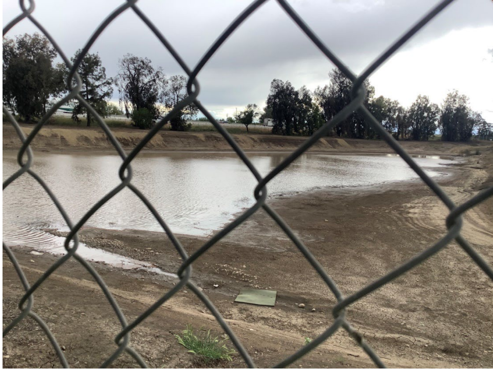
Photo 7. Upland detention basin at corner of Ashby Road and Cooper Avenue, looking west. May 2, 2023.
