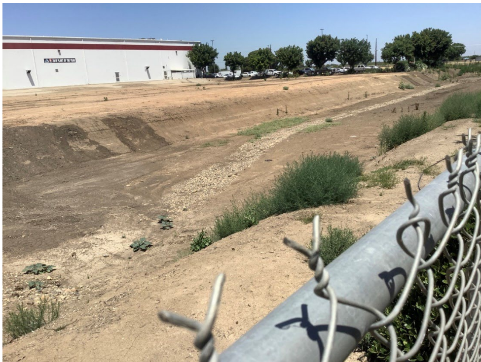
Photo 8. Upland detention basin on west side of Cooper Avenue, looking north. June 13, 2023.
