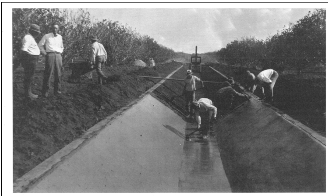
Figure 7. Concrete lining of unknown canal in 1930. (McSwain 105)
