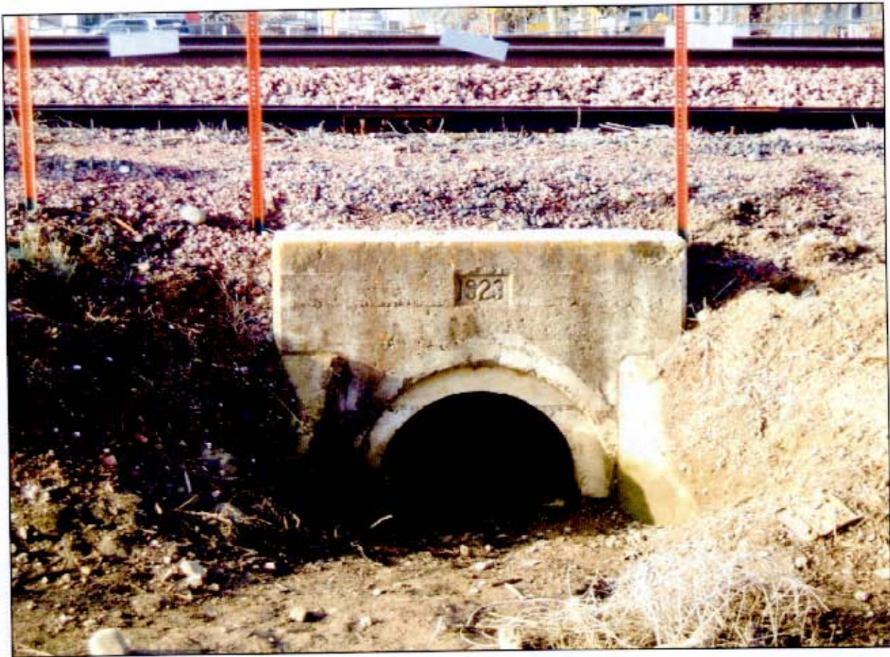
Concrete culvert with date stamp of 1923 (MP 1041.5)
