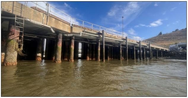
Photo 4. Closer detail of piles under the trestle including sheetpiles which form the breakwater to protect the current boat basin.
