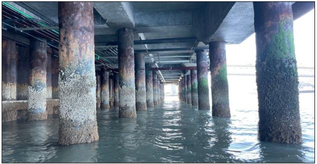
Photo 5. Beneath the main pier. The deck above is solid concrete to allow for heavy equipment and vehicles to load and unload cargo from the TSGB. A similar deck will be necessary for the new pier under the Proposed Project.
