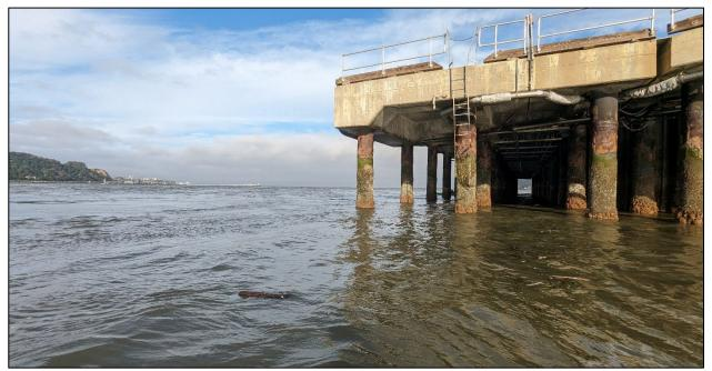
Photo 7. Looking westward along the existing main pier where the TSGB would normally be docked. This pier will be demolished with a new, larger pier constructed on the outboard side (left).
