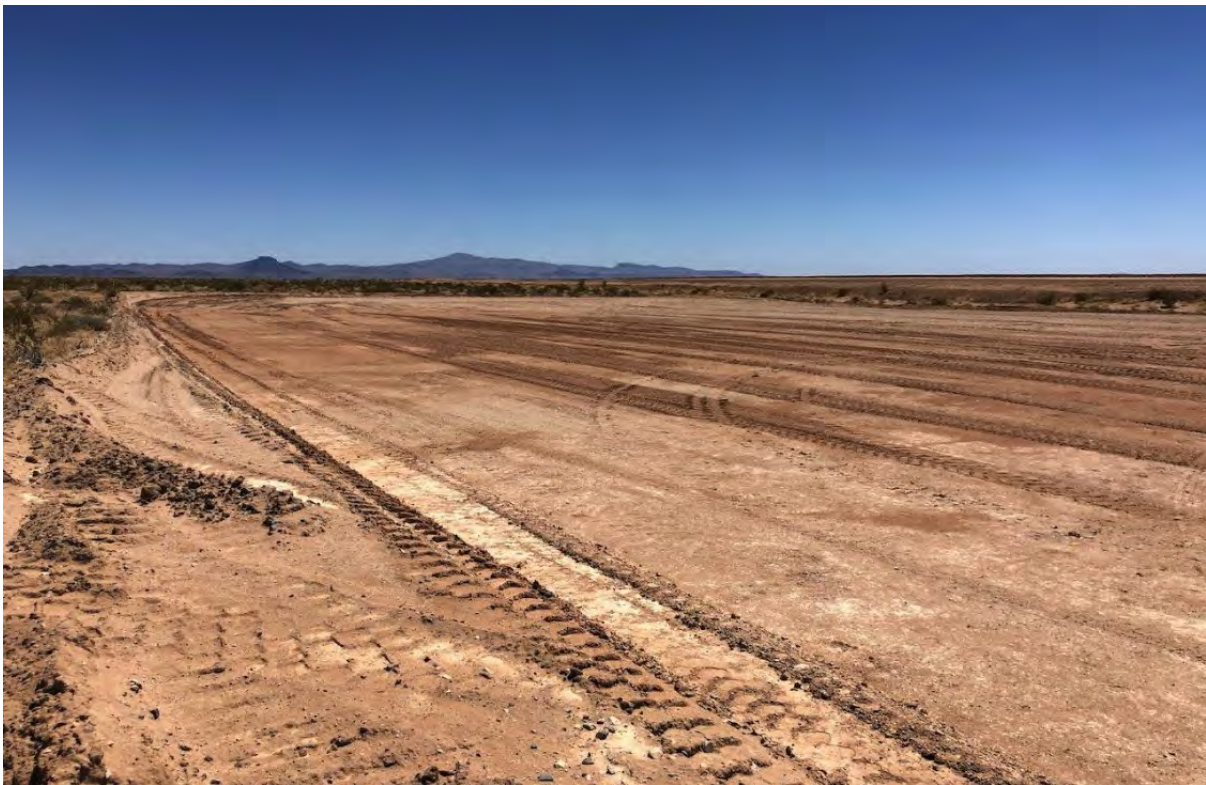
Photograph 2. Overview of SB-2.
