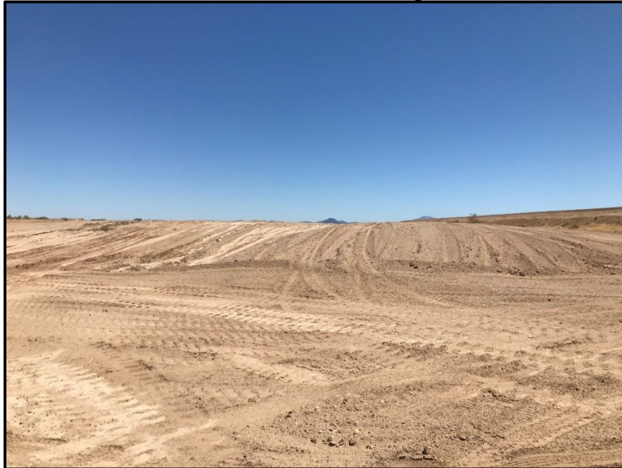
Figure 1.6-3. View of Borrow Site SB-3, View Facing Northeast
