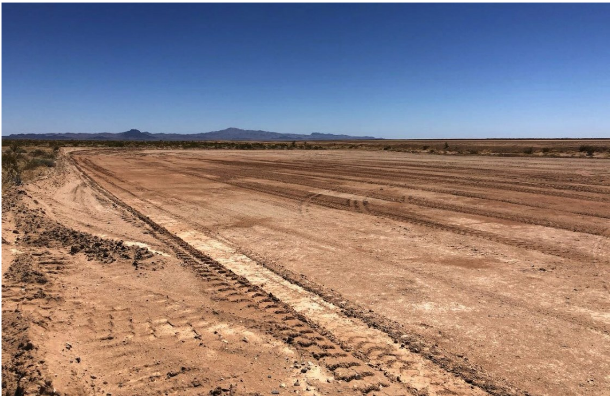
Photograph 2. Overview of SB-2.
