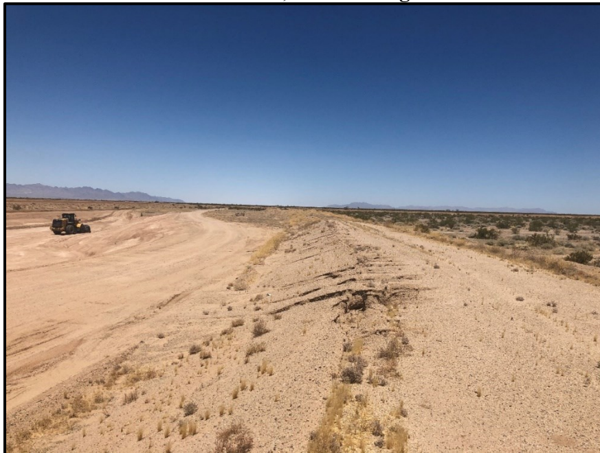
Figure 1.6-4. View of Borrow Site SB-4, View Facing Northwest
