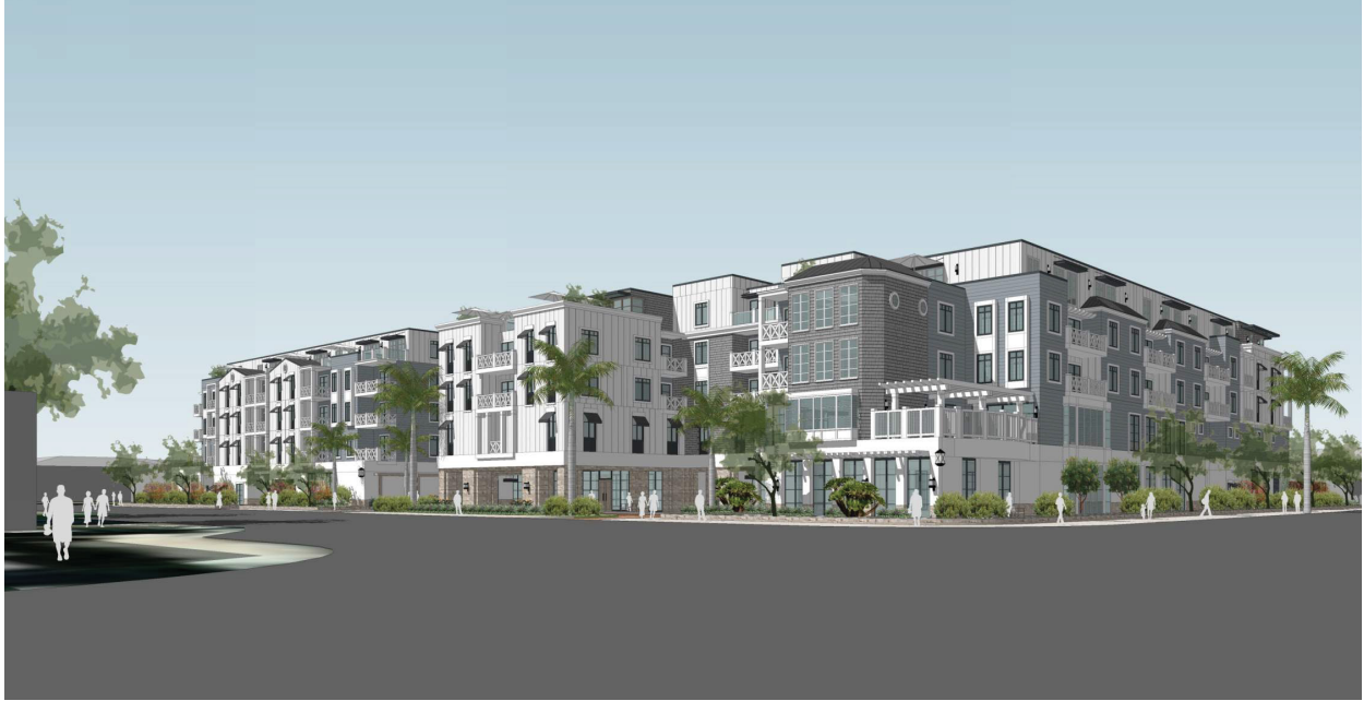
Originally Proposed Project View Southwest from Intersection of Bolsa Chica Street & Warner Avenue
