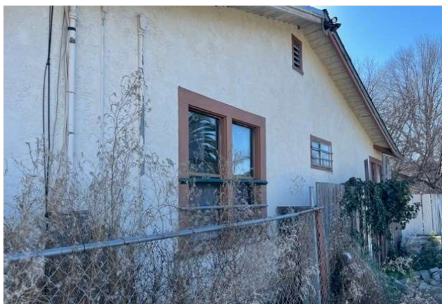
Photo 4: Residence, W elevation, looking SE.
