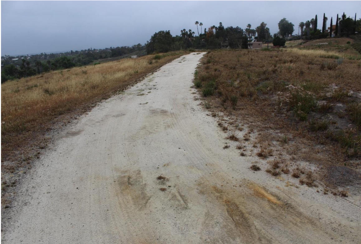
Photograph graded access road with material base on it within Project site. Eocene Sediments visible. View to the west.
