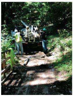
Photograph 2. B-2, west of bridge, drilled with Simco 2400 SK-1
