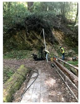
Photograph 1. B-1, east of bridge, drilled with a portable rig
