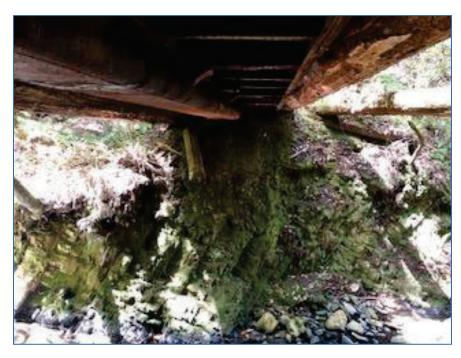
**View 4.** View of underside of existing bridge, showing old railroad car understructure.
