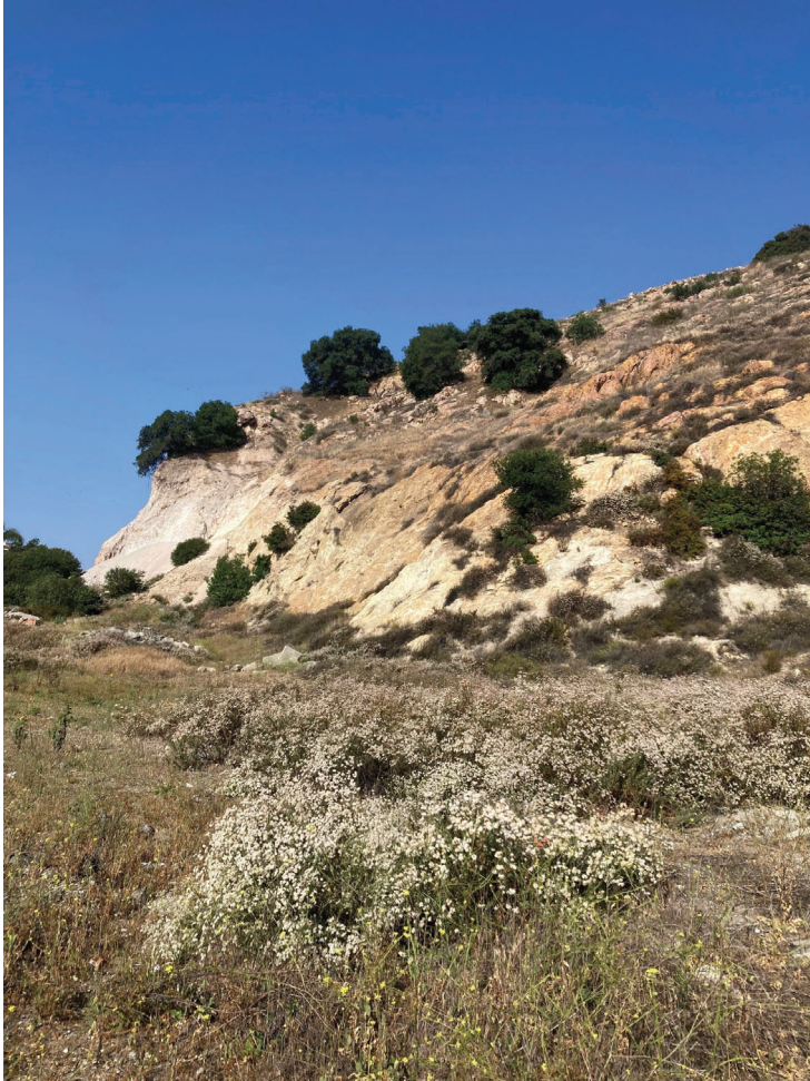
Photograph 3 – View of steep terrain and general tree locations.
