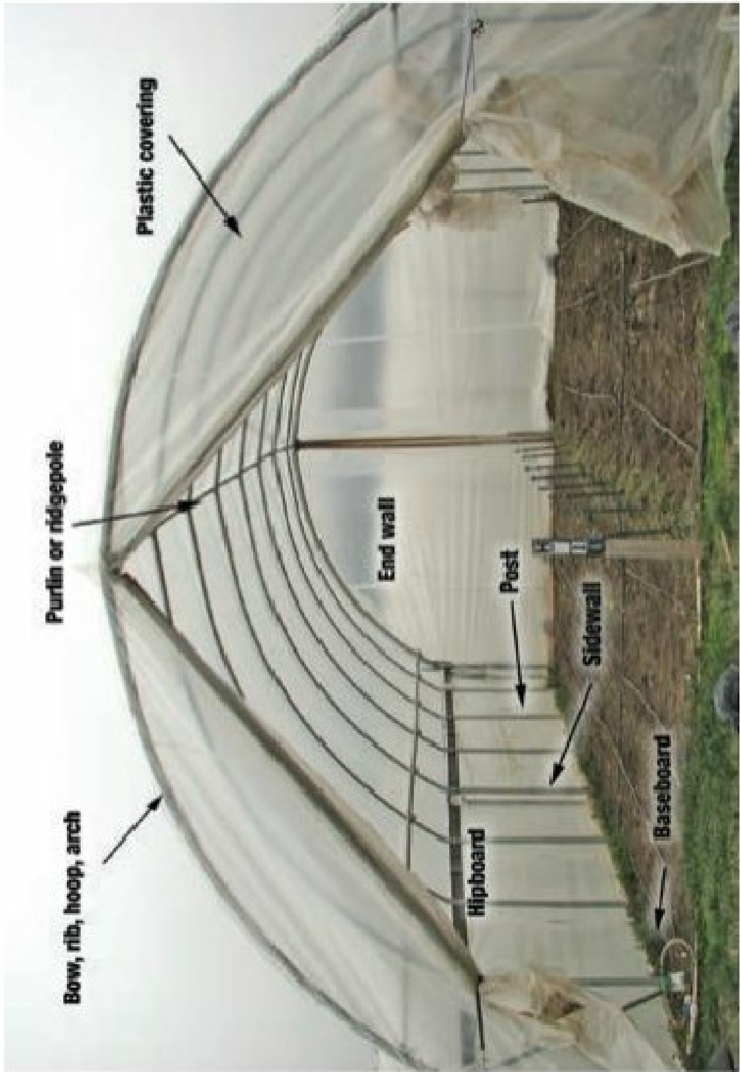
Anatomy of a high tunnel.
