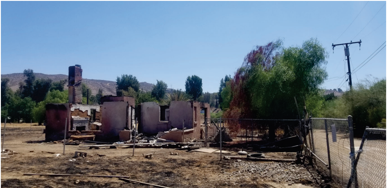
Photo 2: Northwestern portion of the project site, facing south.
