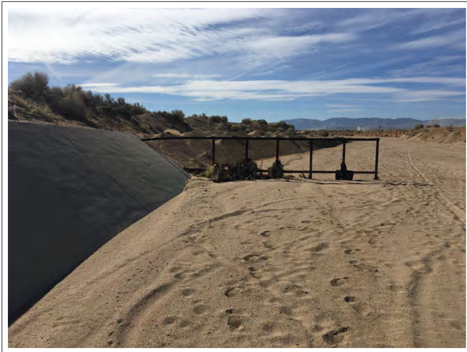
Photo Location 1, March 17, 2022. View of Amargosa Creek, facing upstream. Hardened eastern bank of Amargosa Creek can be viewed near northern end of project site. Trash rack extends into creek.
