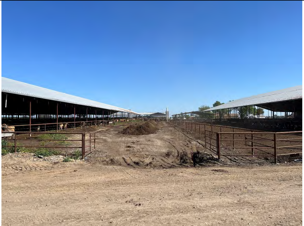
Photograph E. View of area of proposed free stall barn adjacent to existing free stall barns at the South Dairy Facility. View northwest (photograph taken 5/10/2023).
