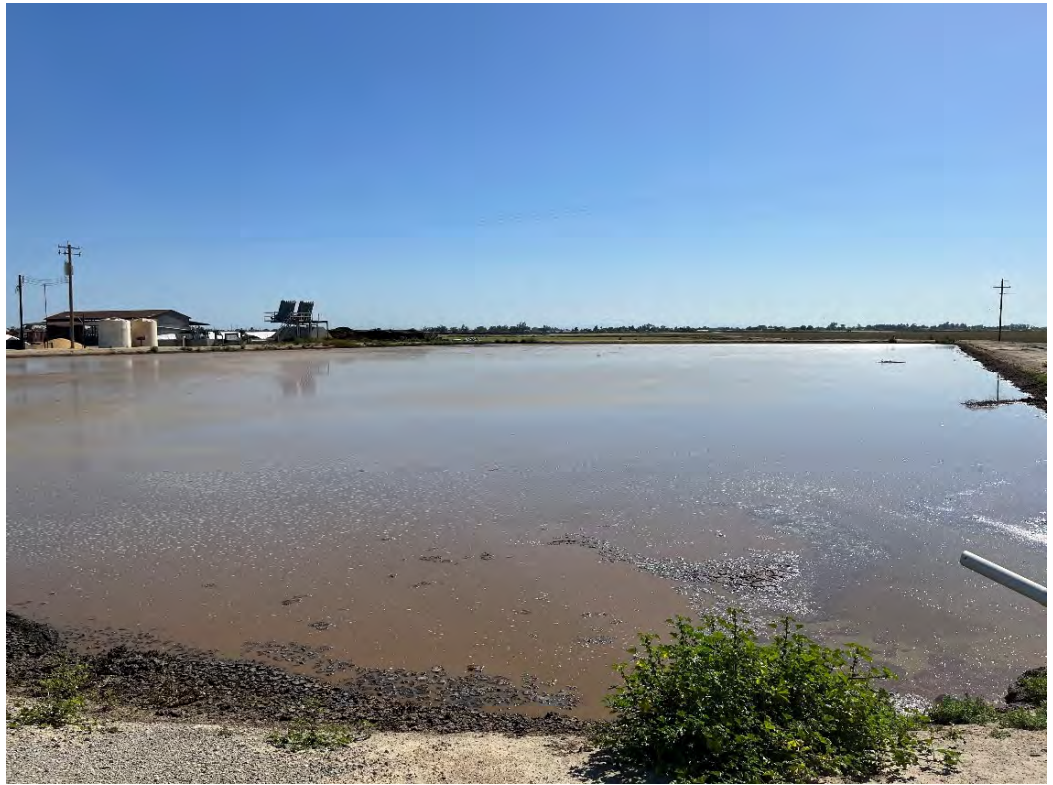
Photograph G. View of existing wastewater pond at the South Dairy Facility. View northeast (photograph taken 5/10/2023).
