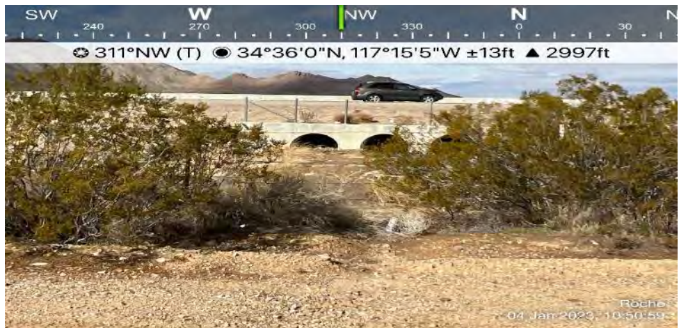
Photograph # 22. Equalizer Culvert under I-15. Water did not leave the Caltrans right of way during the December 2022 through January 4, 2023 storm events.
