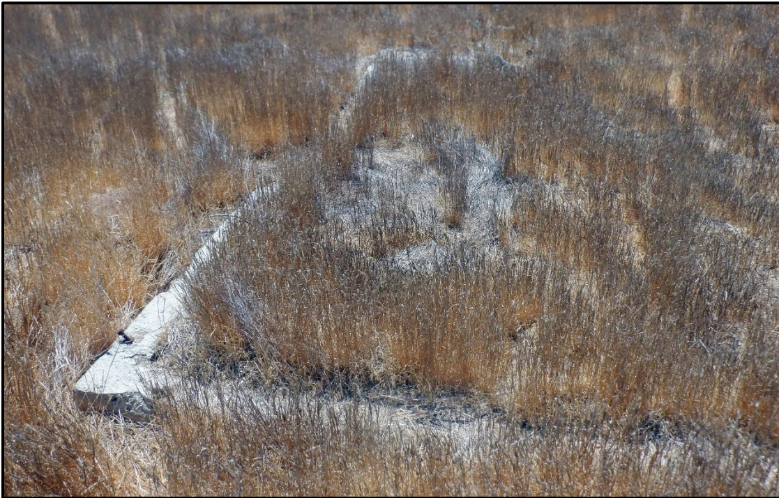
Figure 22. Concrete Foundations Northwest of Main Complex (NW).
