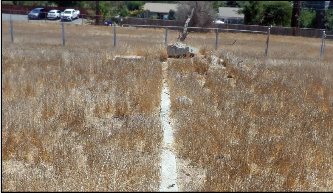
Figure 21. Concrete Foundation running Towards Riverview Drive (SE).
