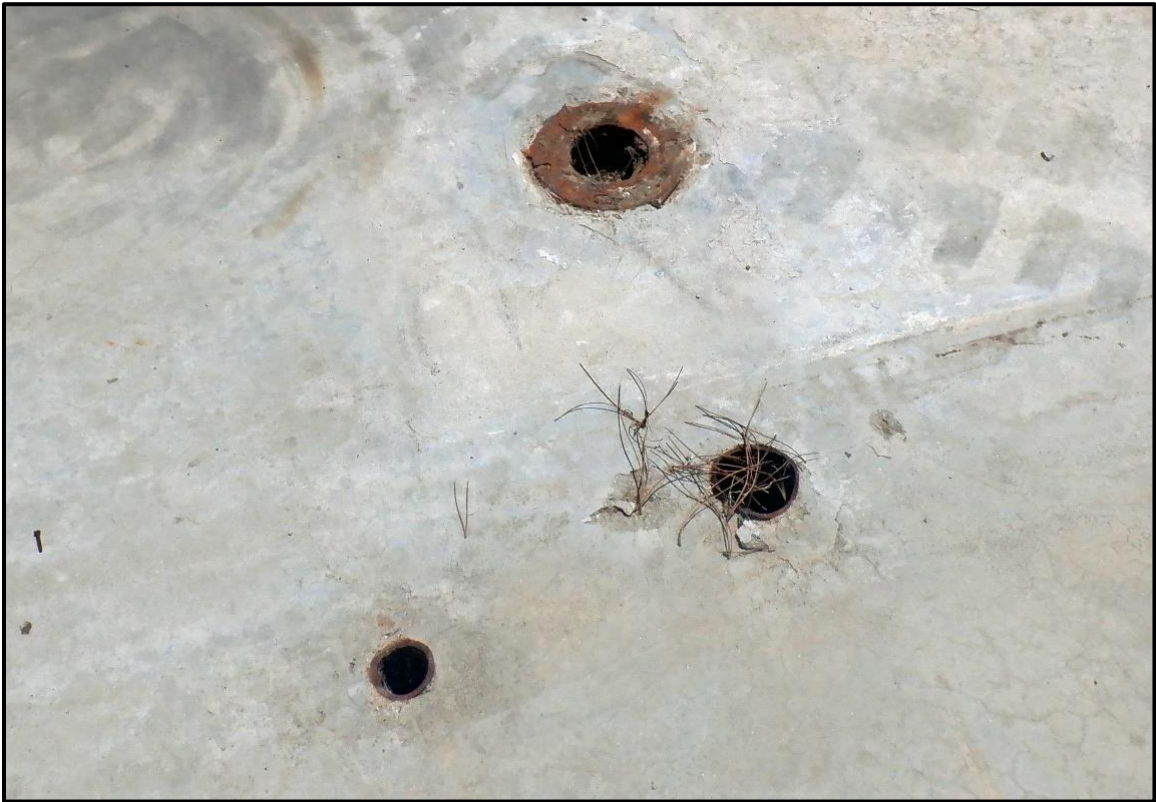
Figure 25. Pipes in Floor of Concrete Slab.
