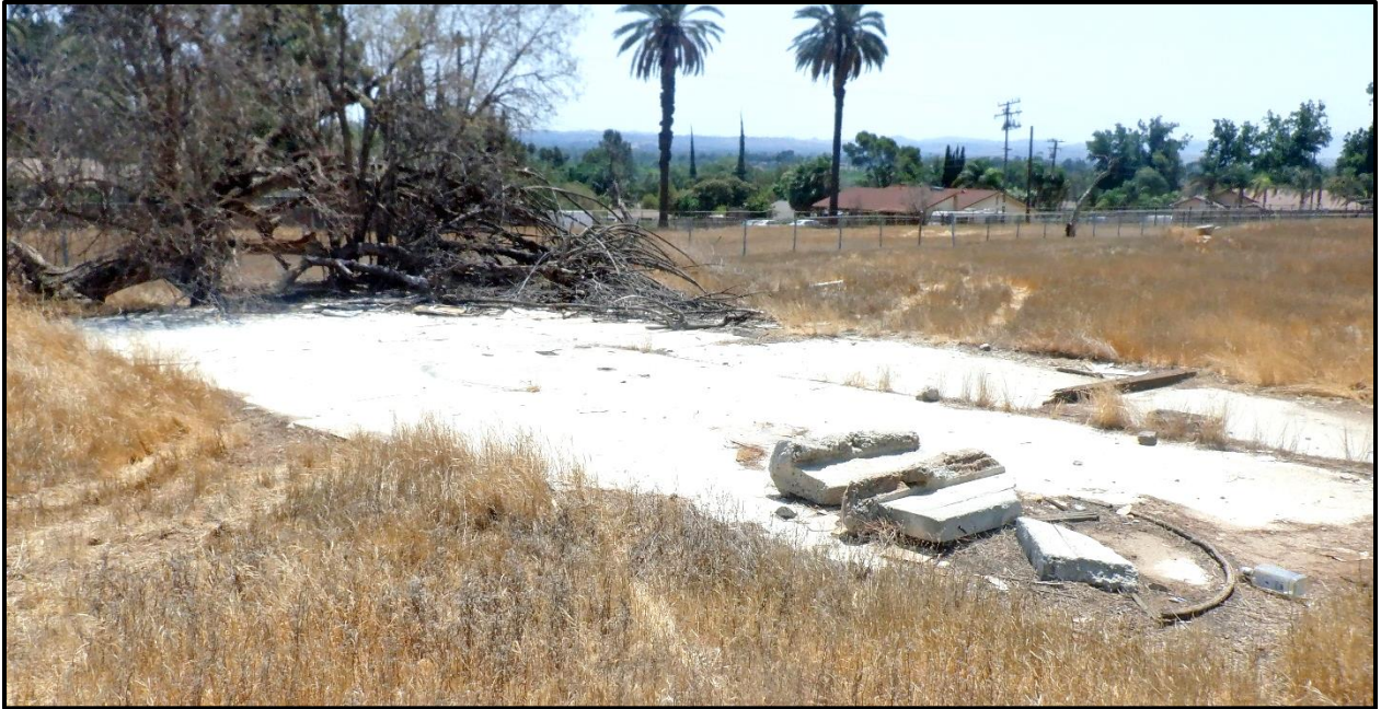
Figure 24. Concrete Slab flanked by Trees and Adjacent to Utilitarian Raised Foundation (SE).
