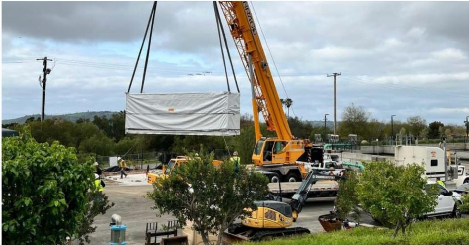
Battery Install at the San Luis Obispo Water Treatment Plant
