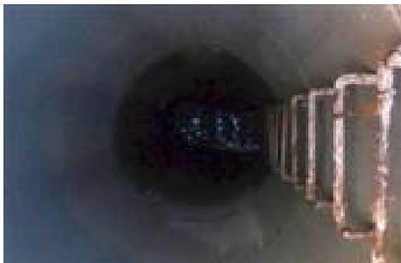
Manhole Before Install
