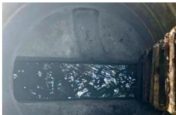
Manhole Before Install
