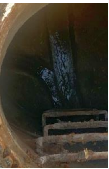
Manhole Before Install
