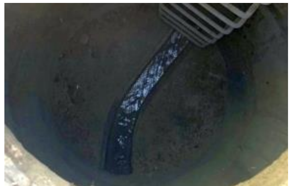
Manhole Before Install
