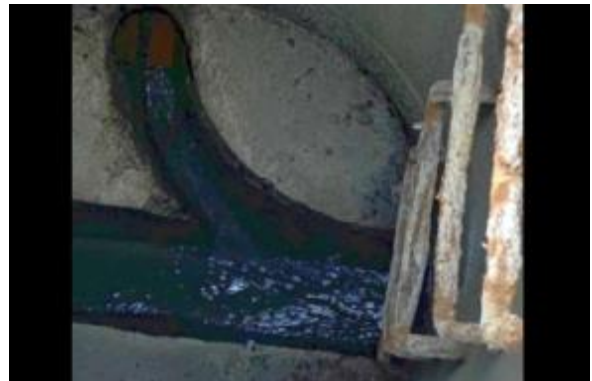
Manhole Before Install
