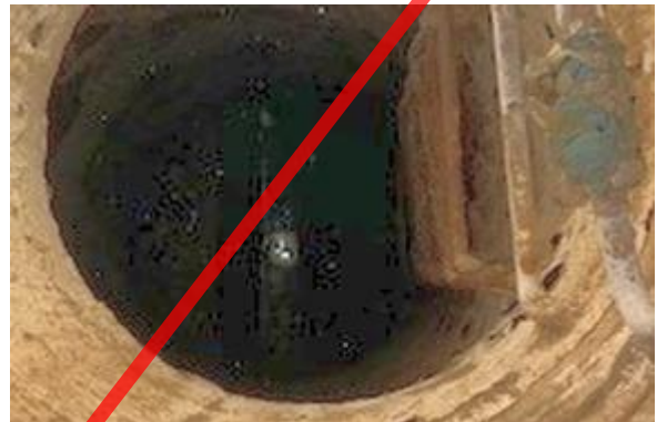
Manhole Before Install
