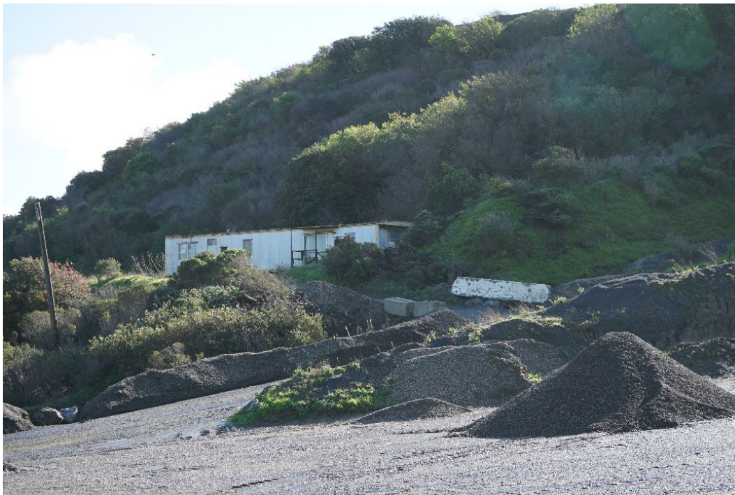
Figure 6-6. Staff Trailer, facing southeast.
