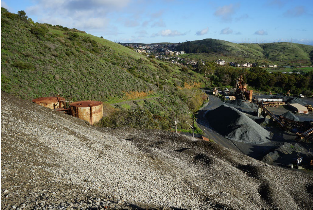
Figure 6-8. Above-Ground Storage Tanks, facing northwest.
