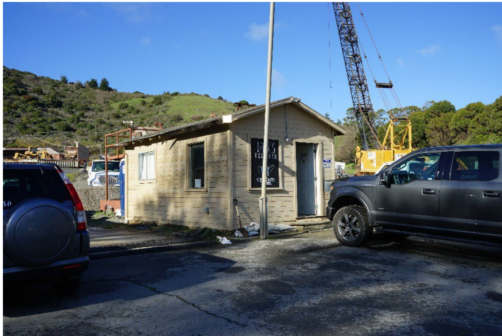
Figure 6-2. Foreman's Office, facing west.
