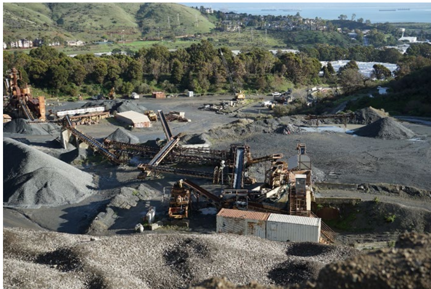
Photograph: Overview of the Primary Crusher & Conveyor Network. View east.
