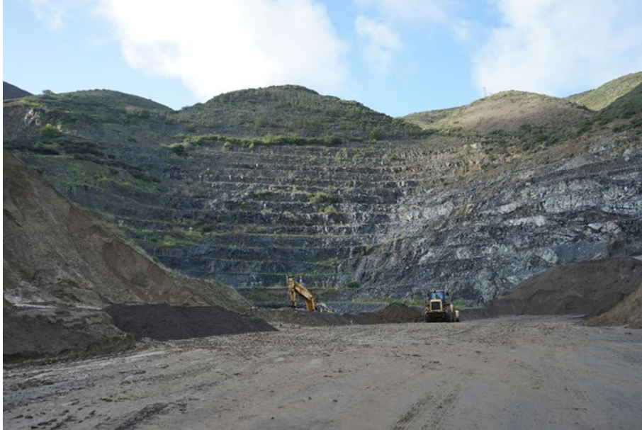
Photograph: Overview of Quarried rock wall. View south.
