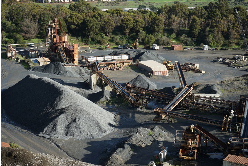
Photograph: Overview of the Processing Yard. View east.
