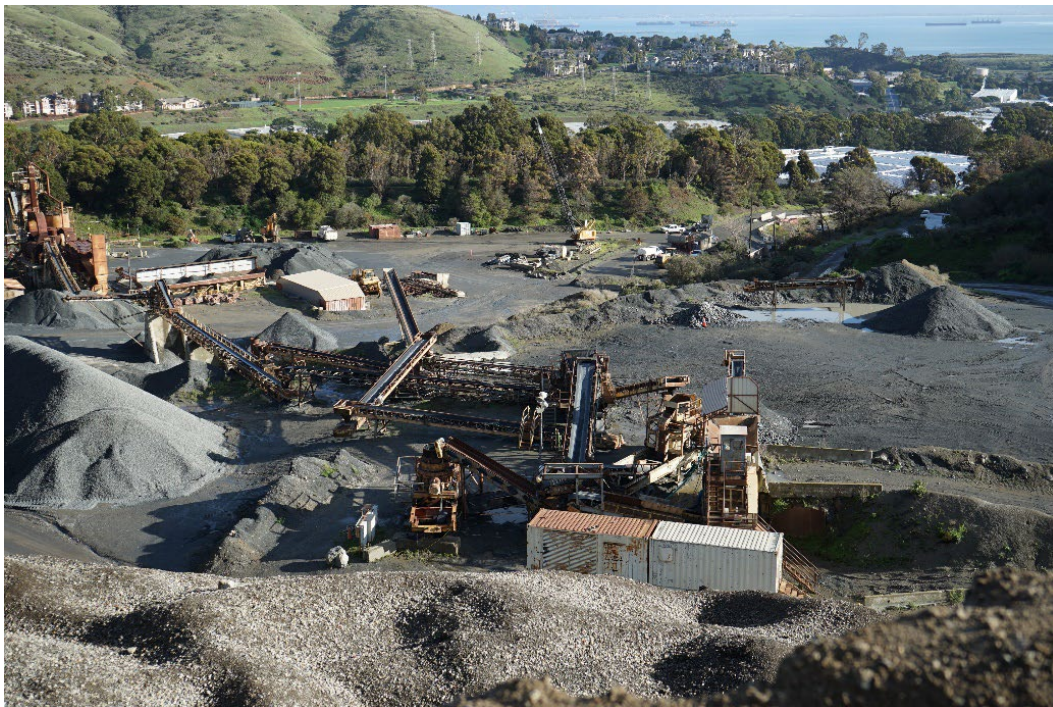
Figure 6-13. Primary Crusher and Conveyor Network, facing east.
