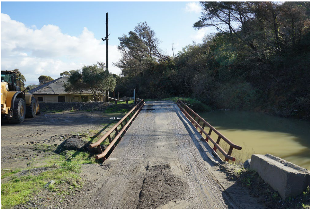
Figure 6-4. Bridge, facing east.
