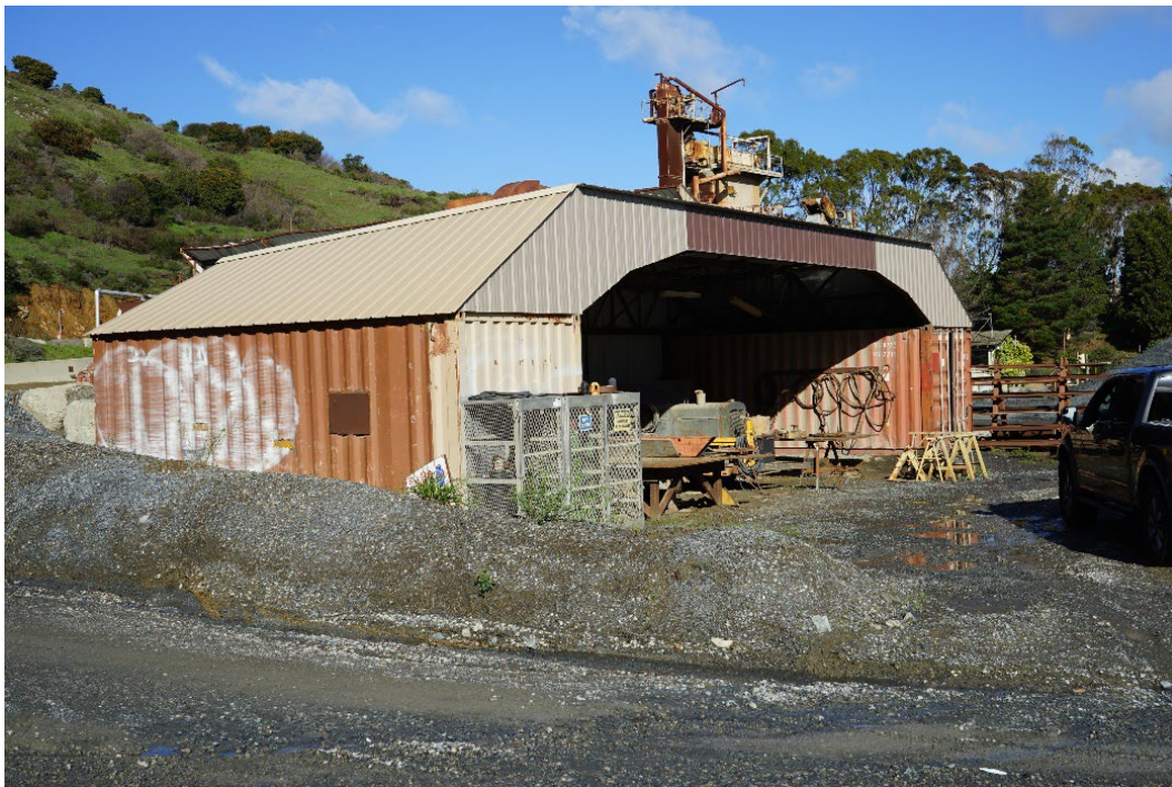
Figure 6-15. Machine Shop, facing northwest.
