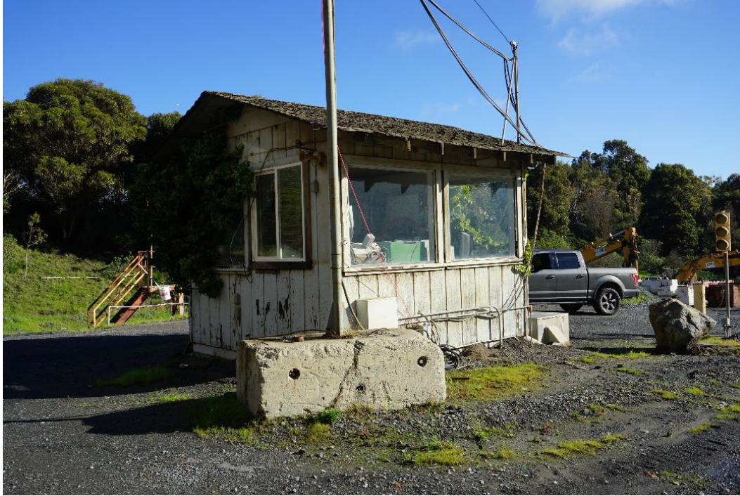
Figure 6-12. Scale House and Scale, facing north.
