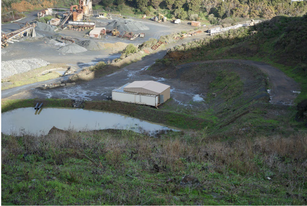
Figure 6-10. Retention Swale, facing north.
