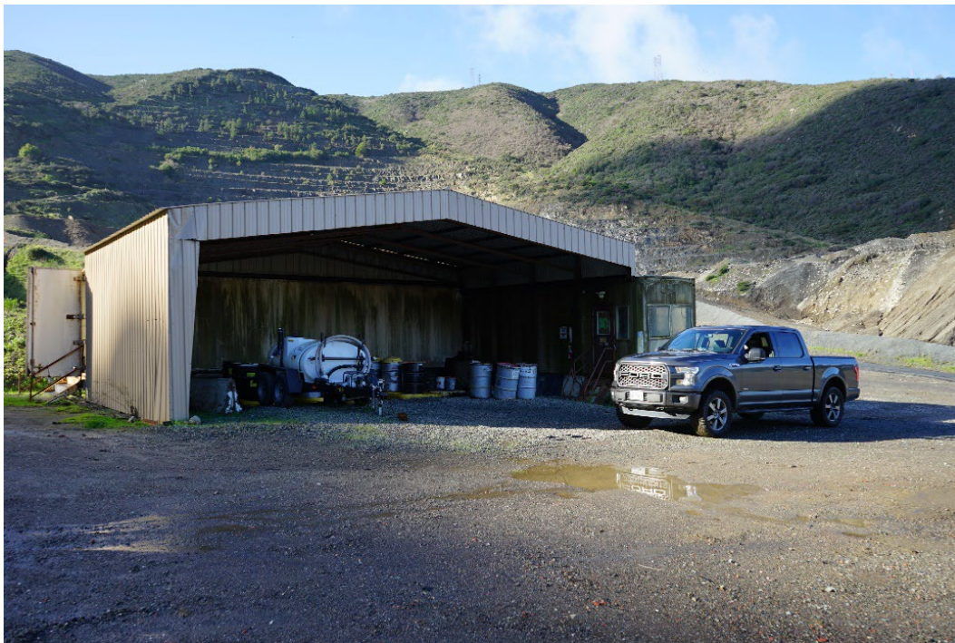
Figure 6-9. Materials Storage Depot, facing south.
