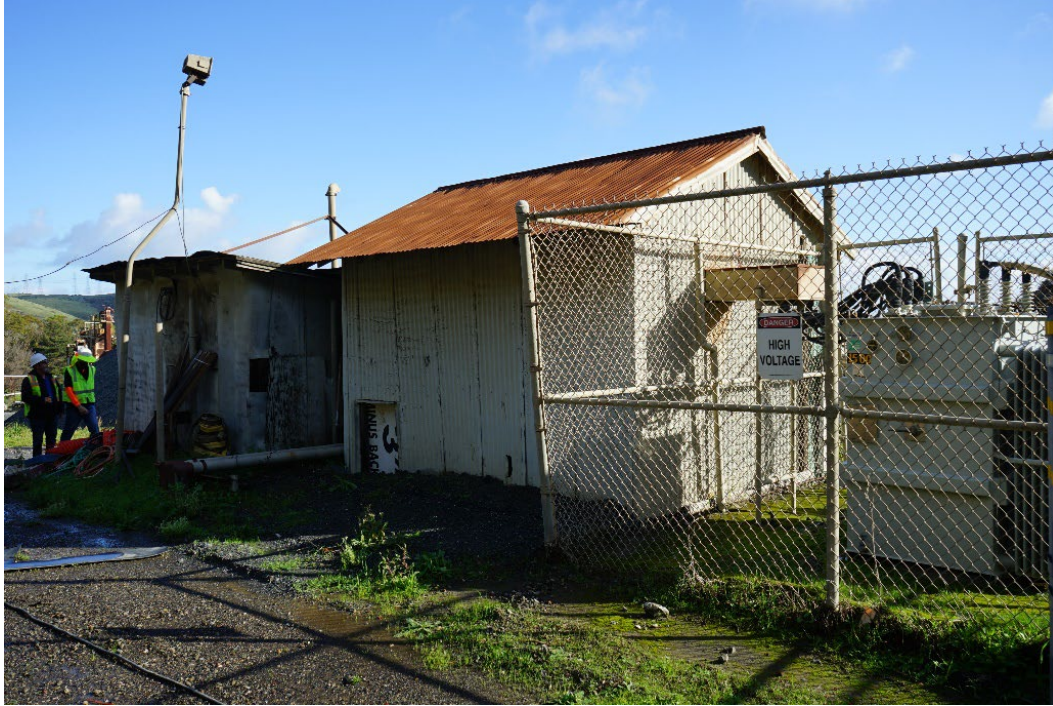
Figure 6-16. Electrical Shed, facing northeast.
