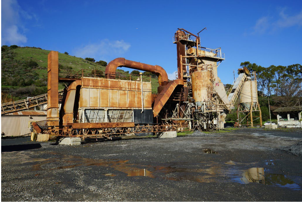
Figure 6-14. Secondary Crusher, facing northwest.
