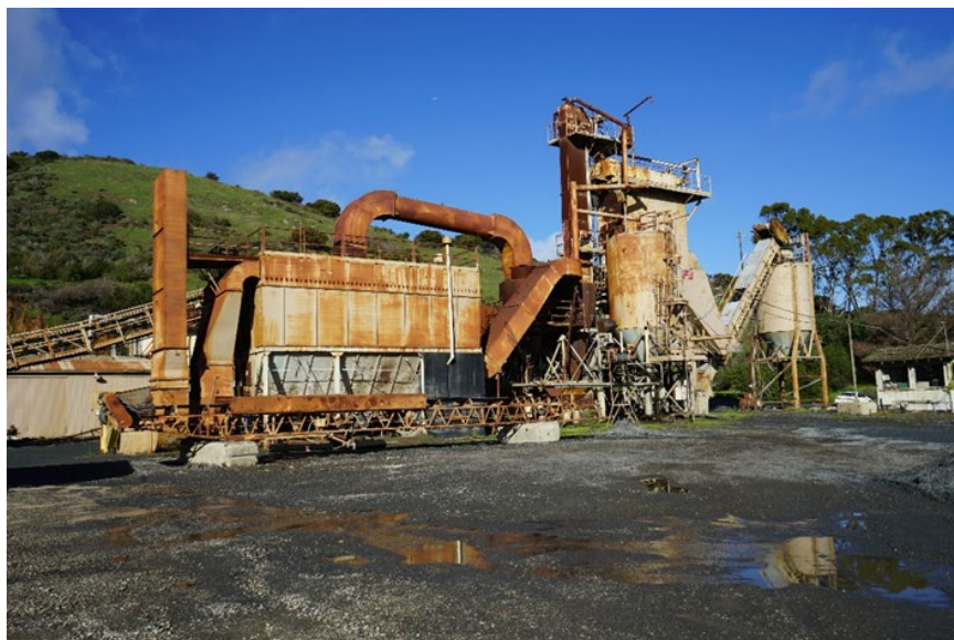
Photograph: Overview of the Secondary Crusher. View northwest.
