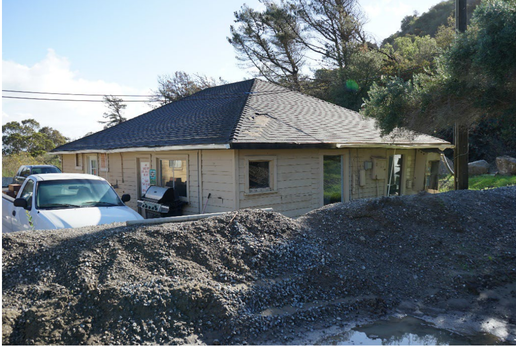
Figure 6-3. Training Building, facing northeast.
