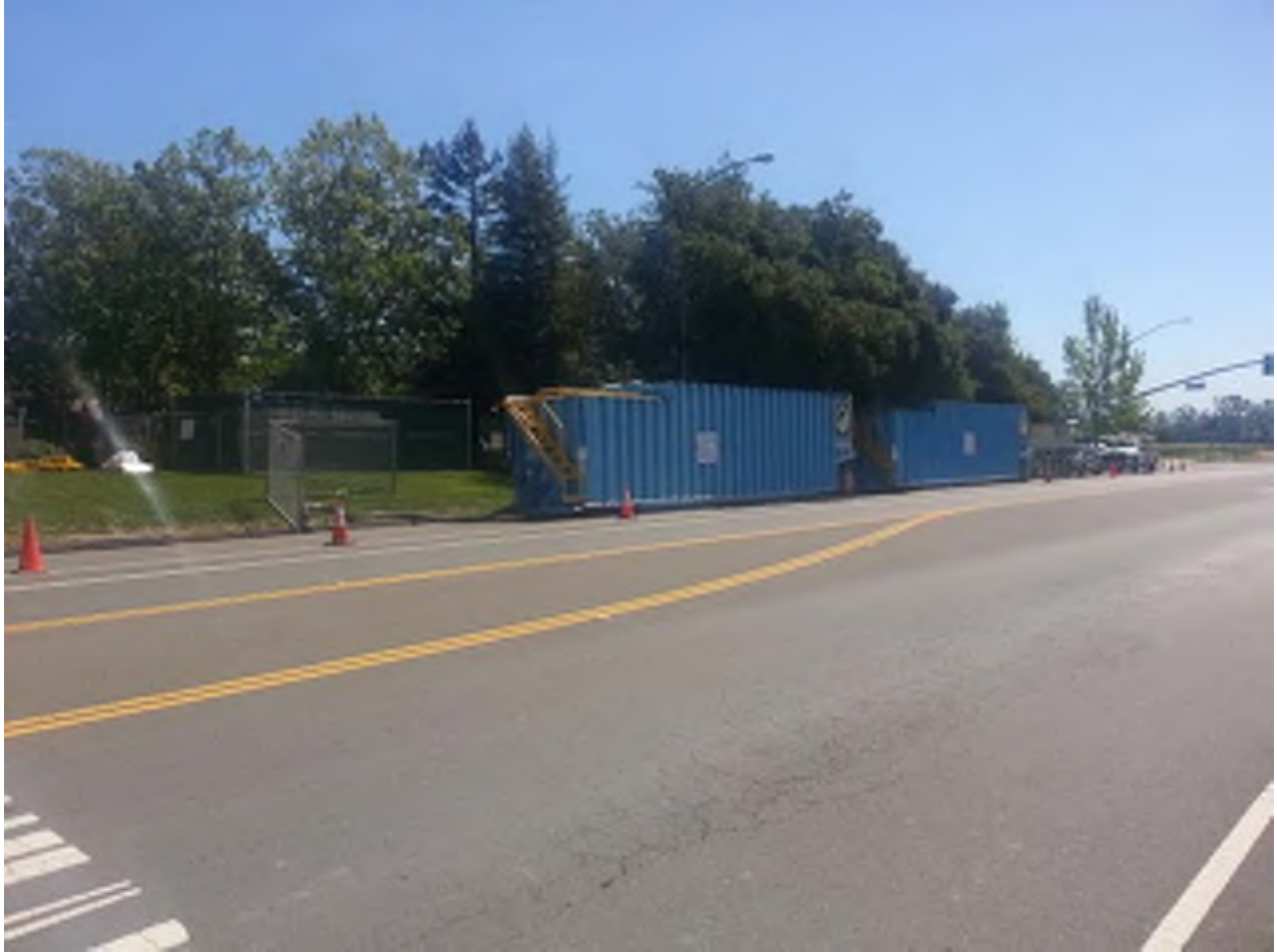
Baker tanks staged along Old Redwood Hwy used for settling of silt prior to filtration through bag filters.
