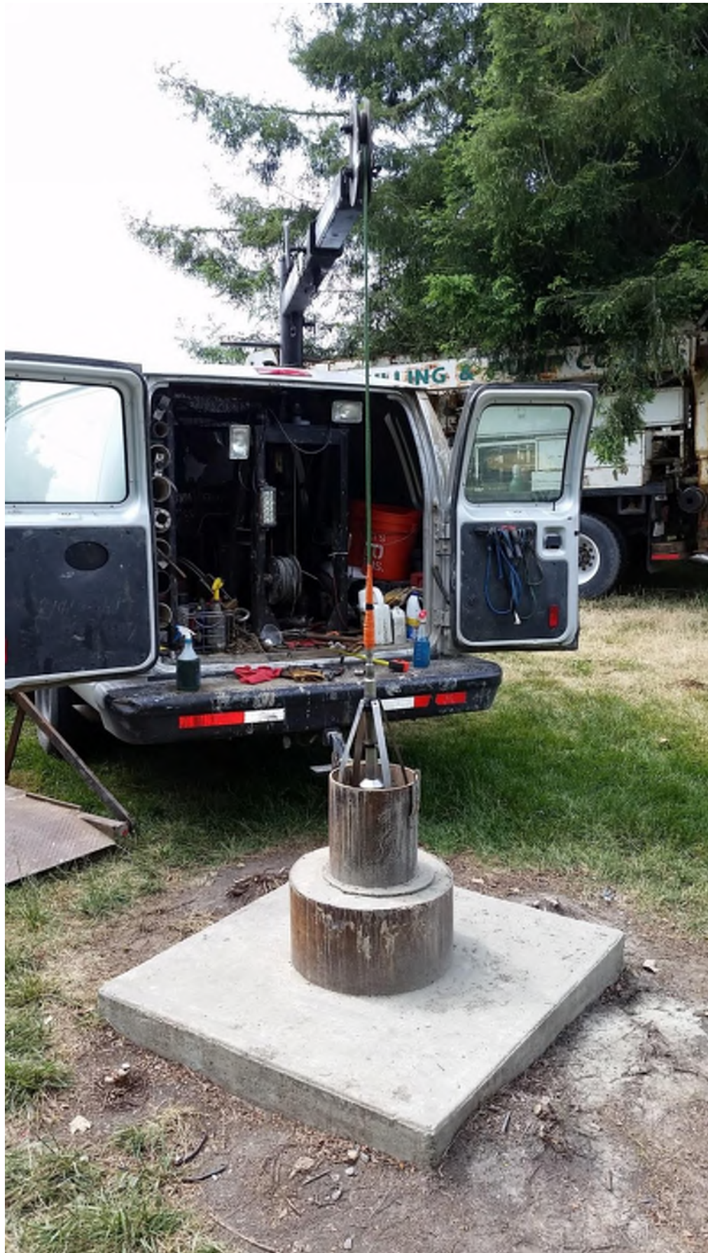
Figure 3 Esposti Supply Well With Camera Tool
