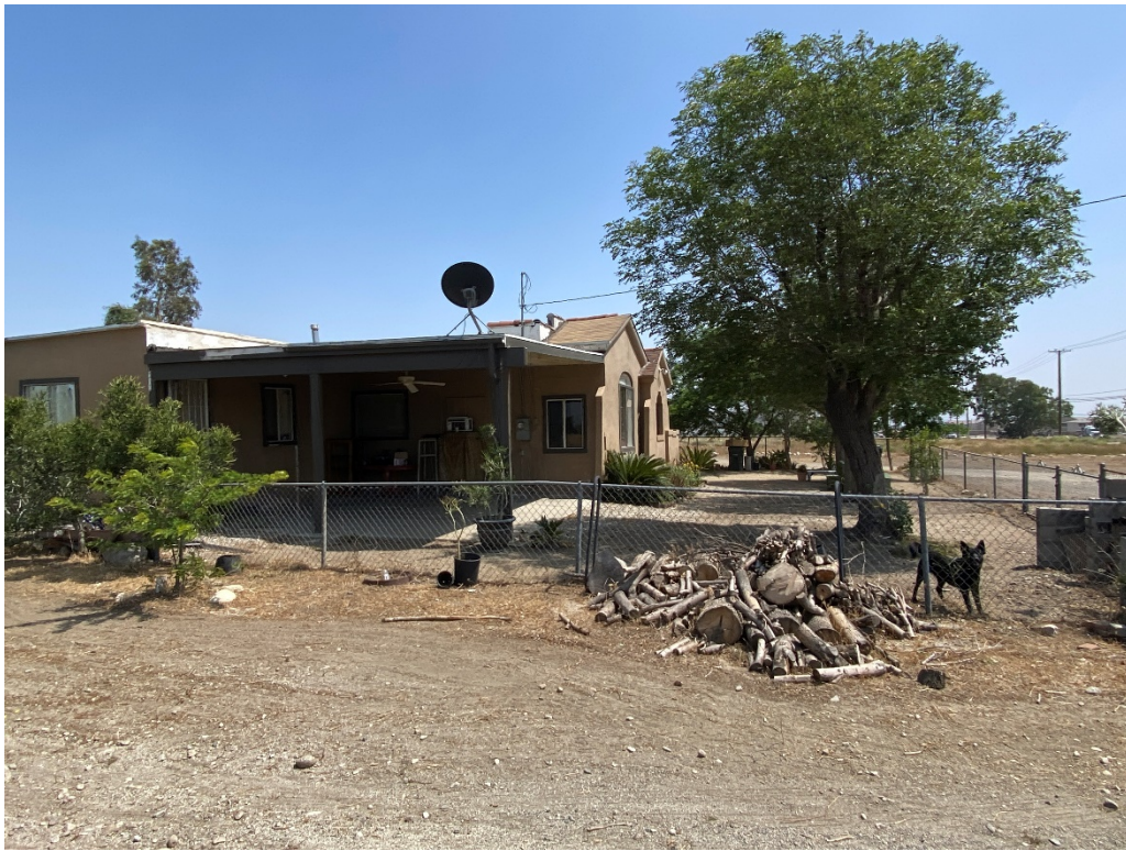
G-11. Residential structure, facing east. (2021-05-19).
