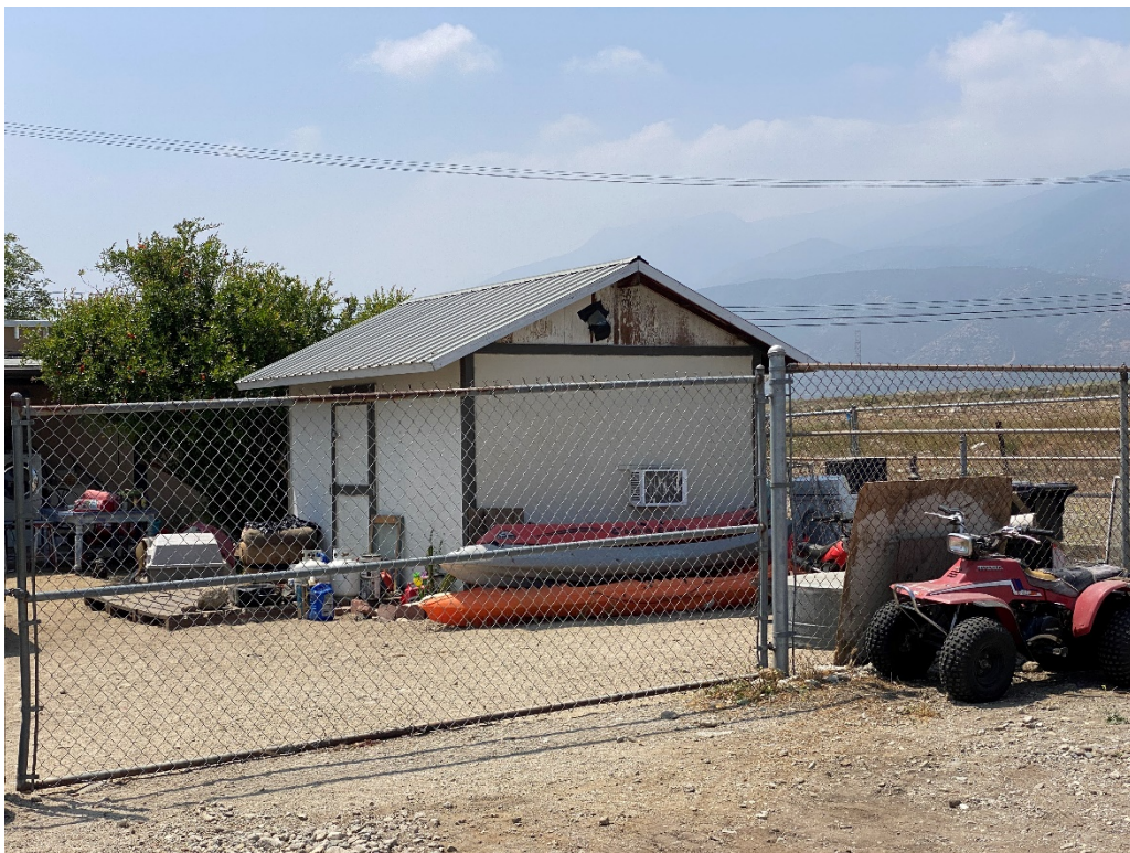
G-12. Shed behind residential structure. (2021-05-19).
