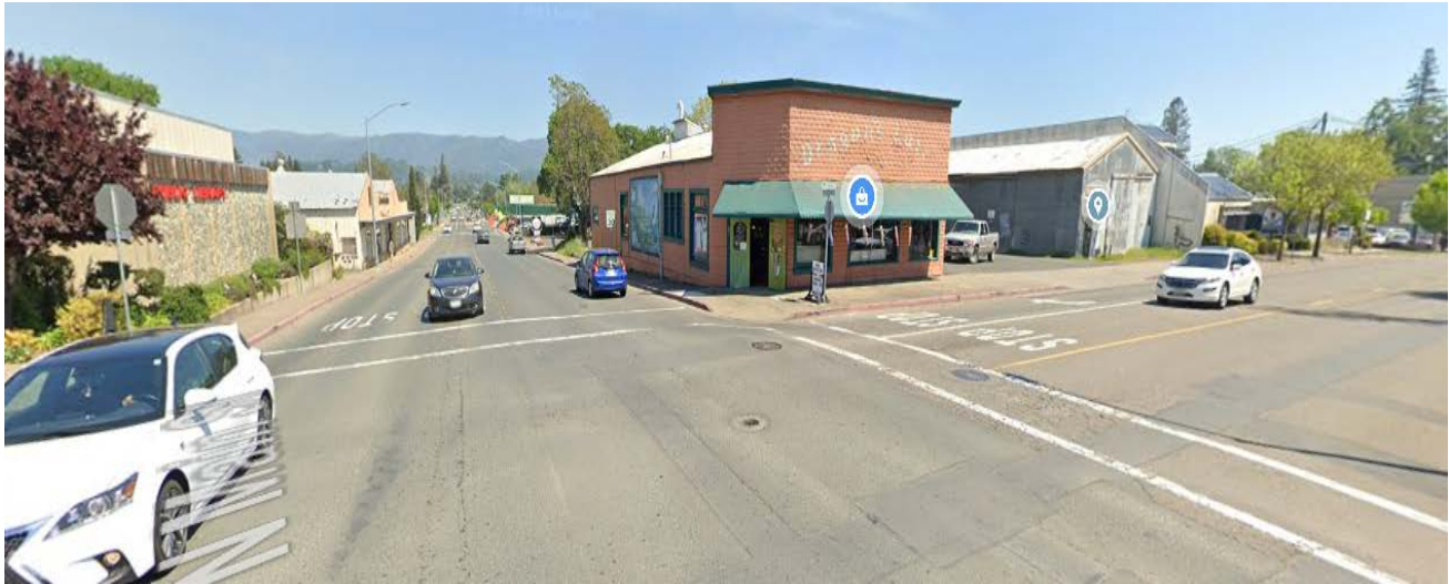
Figure 6, Views Facing East
