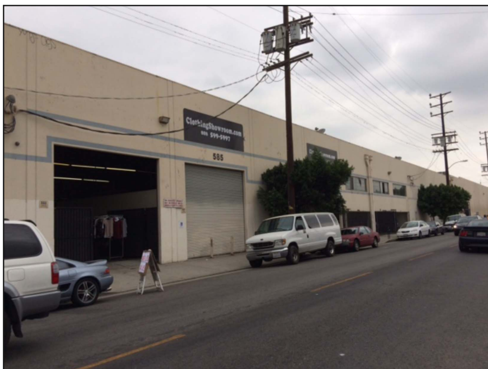
View of the 581-585 Mateo Street property, front elevation, along Mateo Street.
