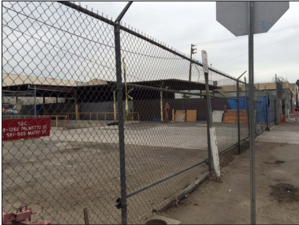
View of the 1260 Palmetto Street property (with flat roof and posts visible) from the intersection of Palmetto Street and Mateo Street.
