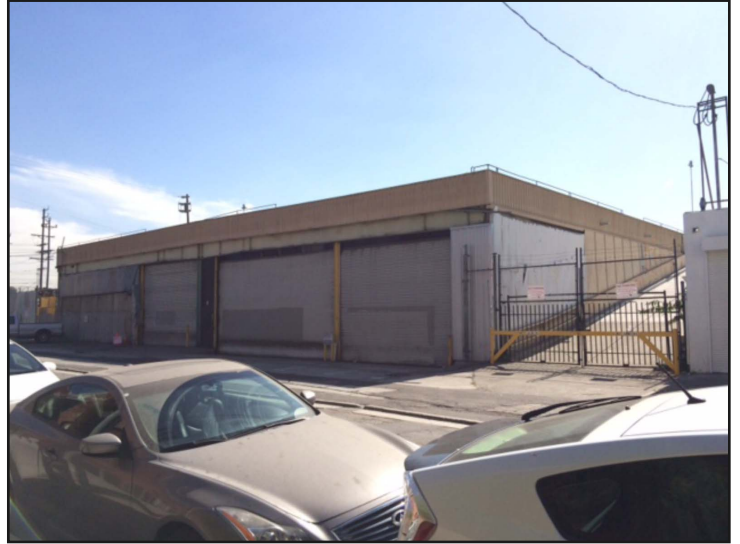
View of the 1262 Palmetto Street property, front elevation, visible from Palmetto Street with associated auto ramp leading to the roof level parking.
