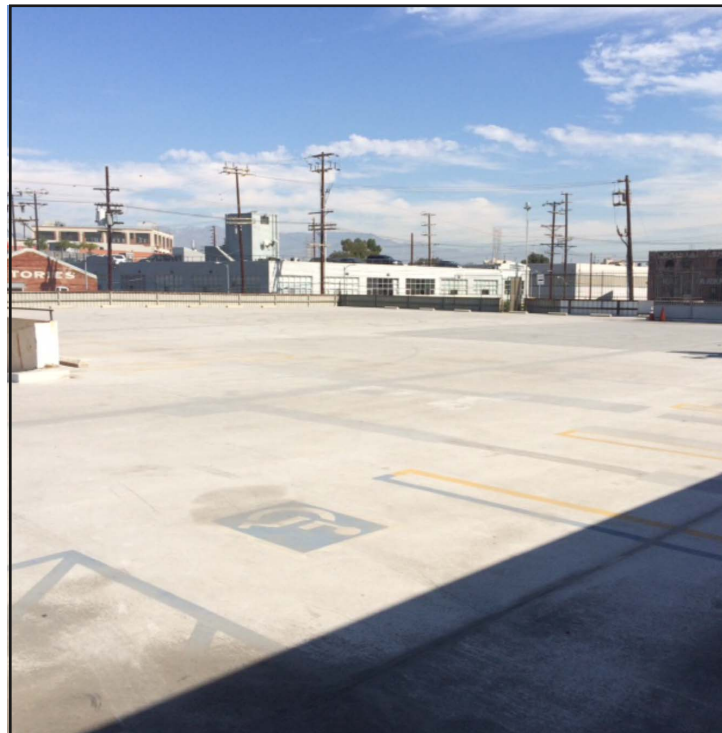
View of the 1262 Palmetto Street property, roof level parking.
