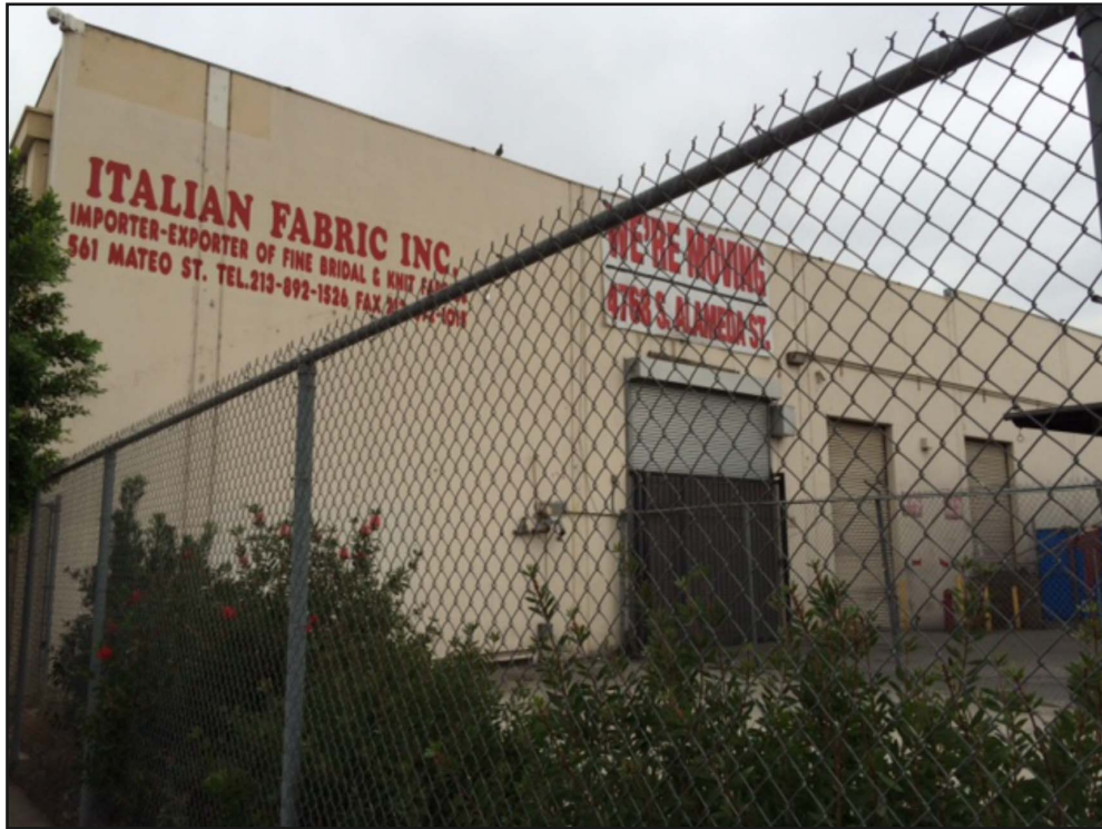
View of the 561 Mateo Street property, front (east) elevation (at left) and north elevation (at right) visible from Mateo Street.
