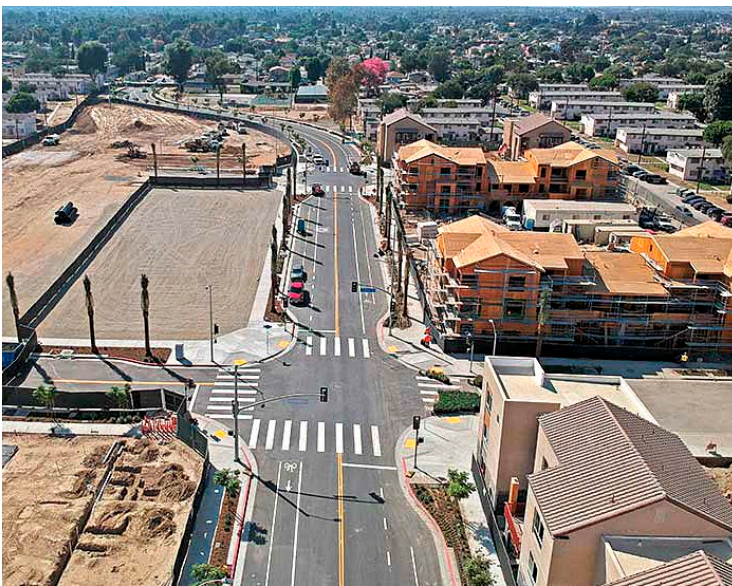
Highway/Bridge - Award of Merit South: Century Boulevard Extension from Grape Street to Alameda Street
