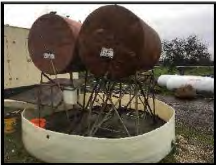
Above-Ground Storage Tanks in Secondary Containment
