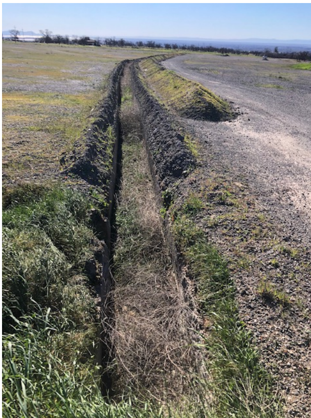
Photo 4. Drain trench cut into gravel clearing.
