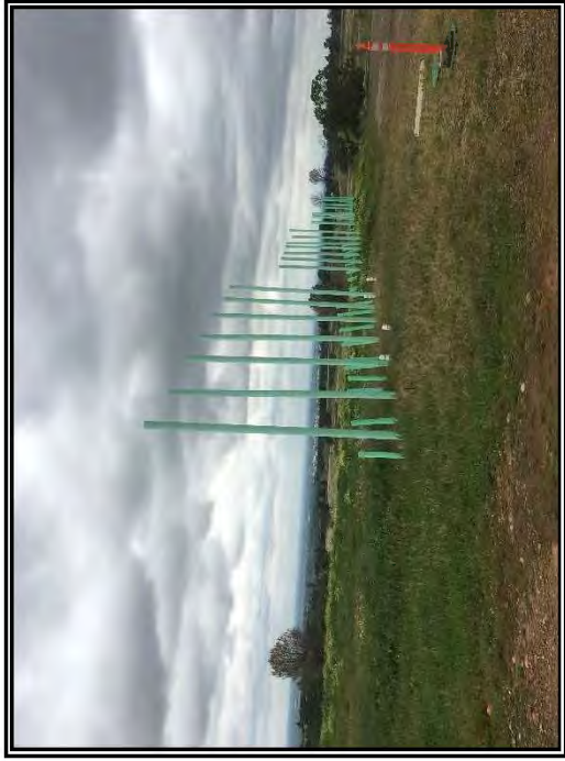
Looking at PVC pipes protruding vertically from the ground associated with a new septic system.
