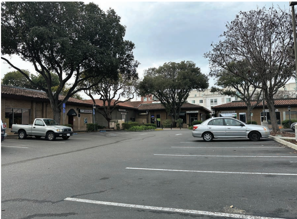
Photo 8: View of existing commercial building looking west from parking lot.
