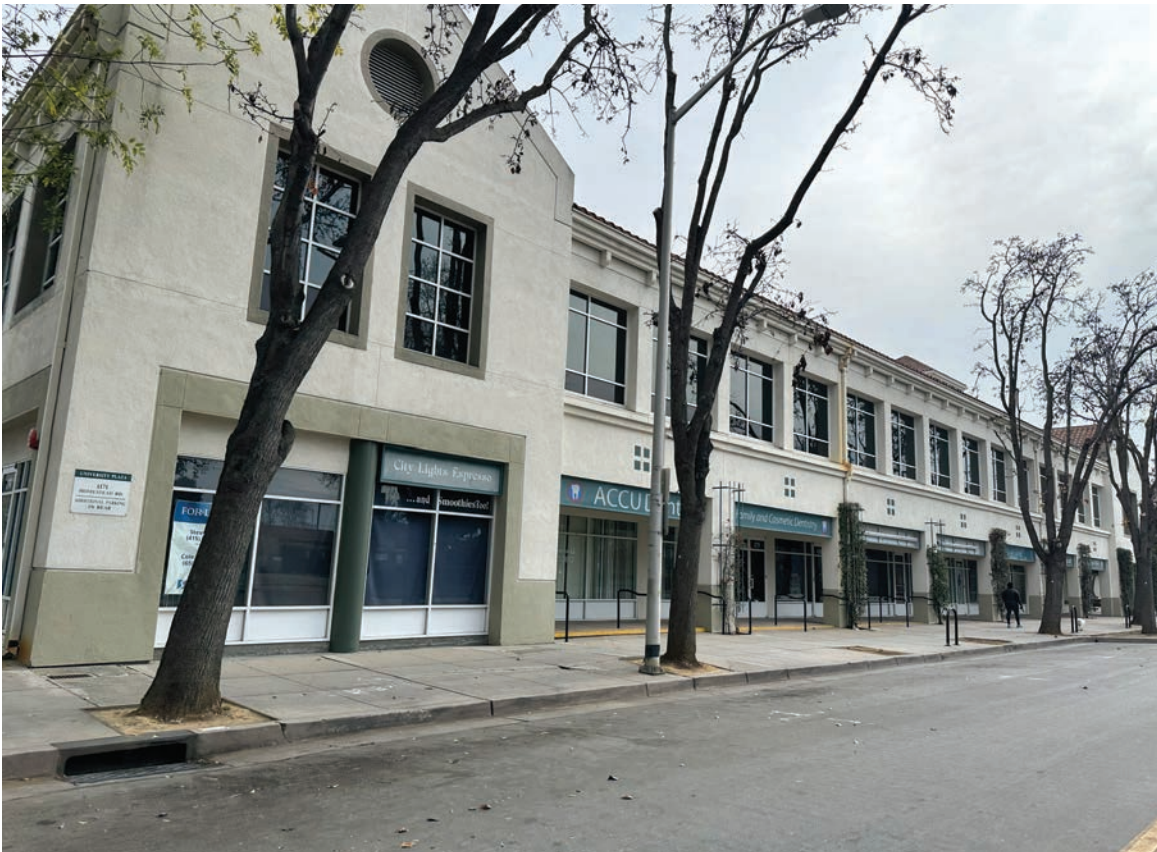
Photo 4: View of existing commercial building looking southeast from Jackson Street.
