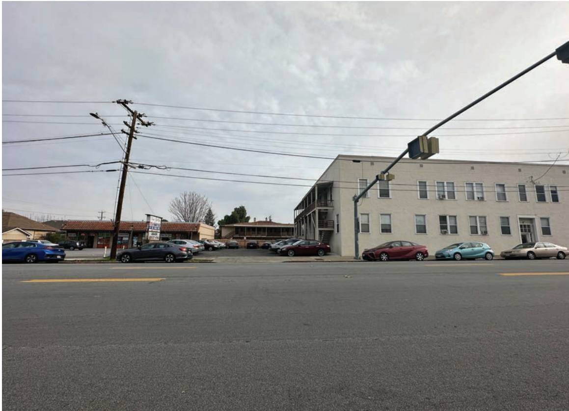
Photo 9: View of existing multi-family residence and commercial building looking southeast of Lafayette Street.
