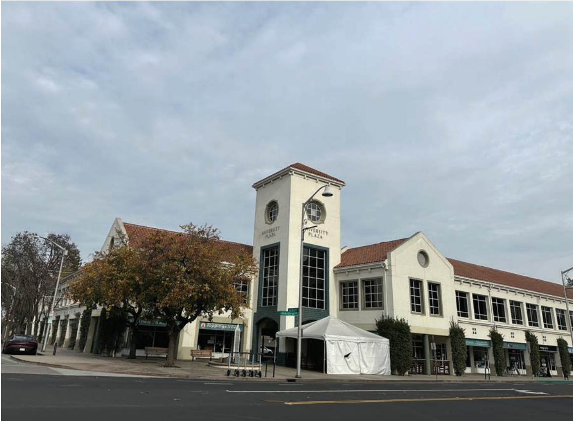
Photo 3: View of existing commercial building looking north from Homestead Road.
