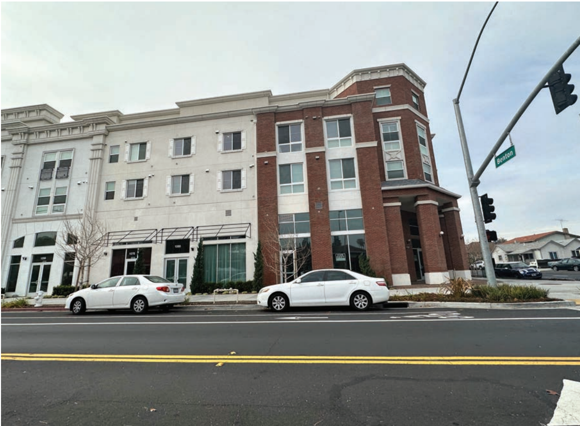
Photo 6: View of existing mixed-use development looking west on Monroe Street.
