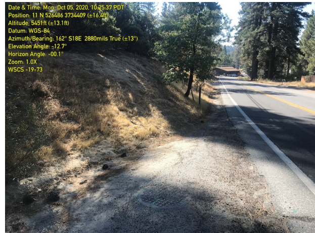
Erosion rill on Parcel 017 where “bowl” area appears to drain toward Highway 243 – prior to grading (10.05.2020).
