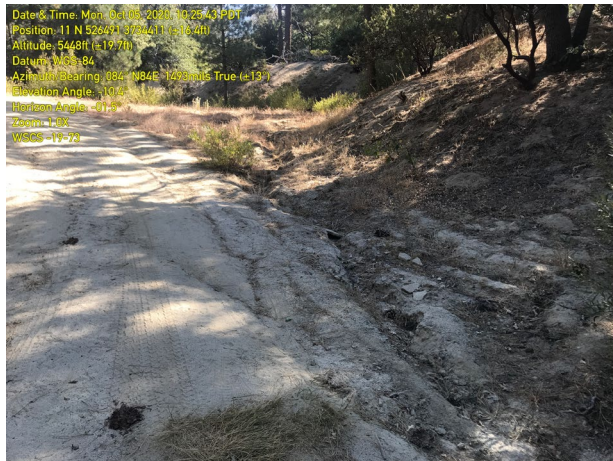
Erosion rill on Parcel 017 where “bowl” area appears to drain toward Highway 243 – prior to grading (10.05.2020).
