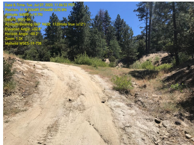
Driveway (south end) on Parcel 017, from Highway 243 looking east-northeast – prior to grading (07.07.2020).
