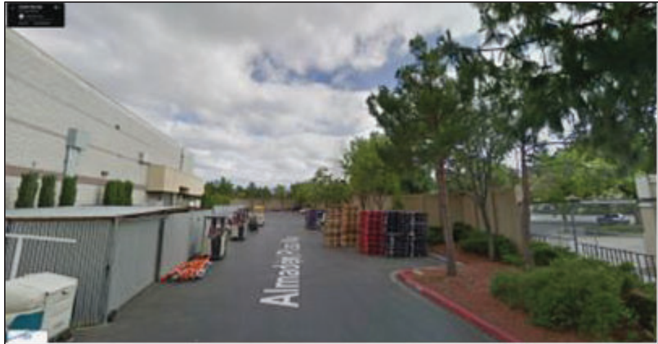
Almaden Costco sound wall separating residential neighborhood.
