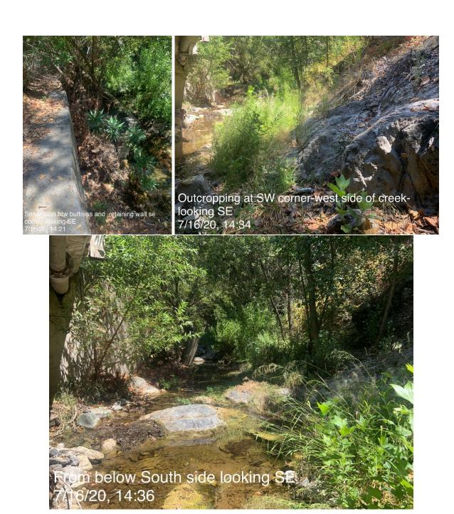
Photo 8. At the southeast corner of the Bridge, there is separation between the buttress and retaining wall (left) and an outcropping along the west side of Silverado Creek (right).
