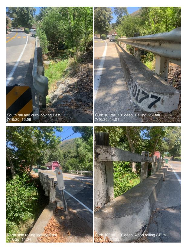
Photo 4. Concrete curbs with metal guard rails and painted wooded posts extend along the south side of the Bridge. Concrete curbs with painted wooden posts and painted wooden guardrails extend along the north side of the Bridge. Yellow and white striping, and botts dots, extend along the north and south sides of the Bridge.
