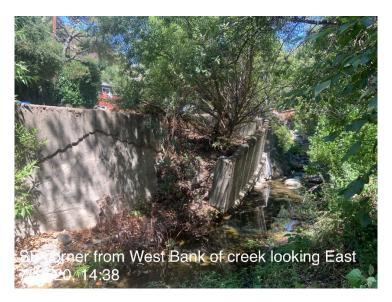
Photo 9. South of the Bridge, looking east; land subsidence occurs at the southeast retaining wall.
