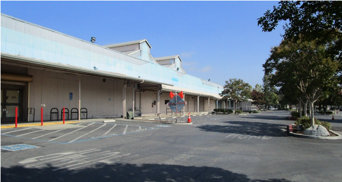
Photo 1. View of existing structure on the project site, taken from the northwest portion of the project site looking south.
