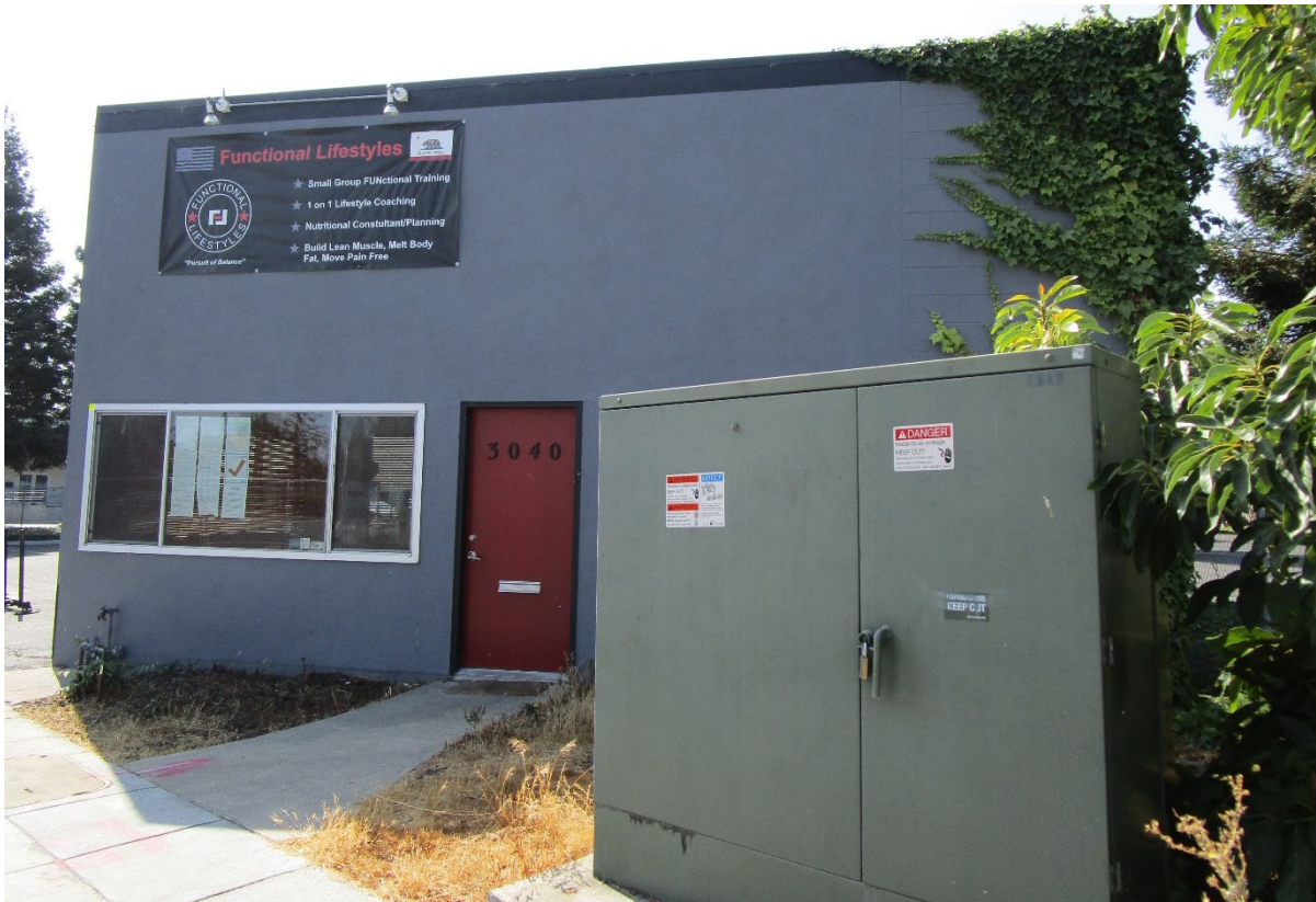
Photo 2. View of existing structure at 3040 Park Boulevard from Park Boulevard sidewalk looking southwest.
