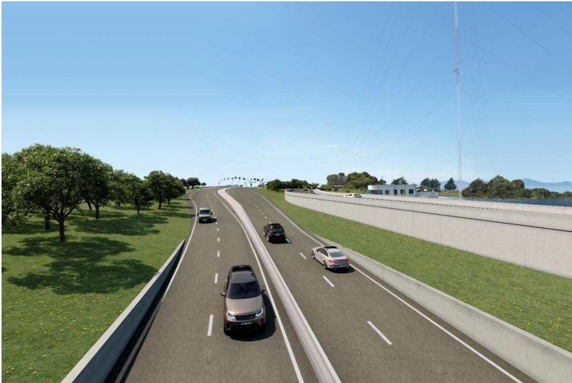
**Proposed Project:** As shown in Figure 2.1-23, the proposed project would add a new Ashby Avenue extension with four travel lanes, extending to the middle of the interchange at intersections connecting with east- and westbound on- and off-ramps to I-80. Ashby Avenue would extend beyond the interchange and connect with West Frontage Road.
